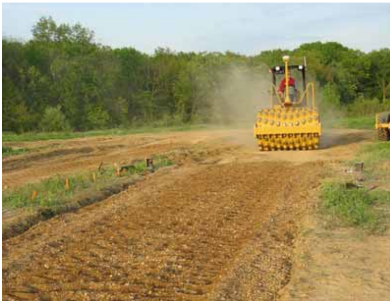
Figure 152. Soil compaction using CP-533 vibratory padfoot roller
