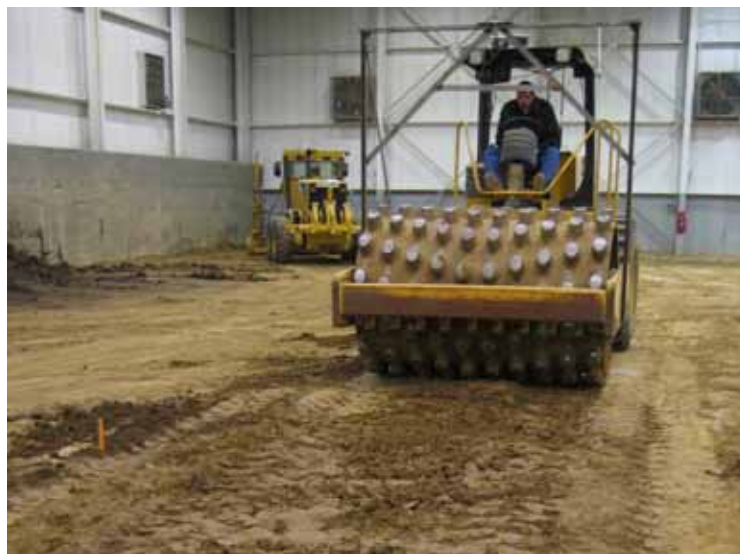
Figure 5. Soil compaction using prototype CP-533 static padfoot roller
