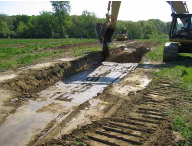
Figure 147. Excavation of test strip
