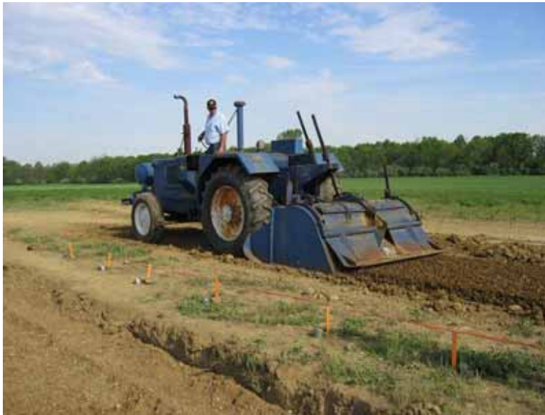
Figure 150. In situ soil mixing using a road reclaimer
