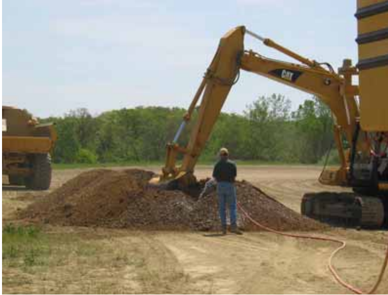
Figure 149. Moisture conditioning of test soils prior to placement in strips
