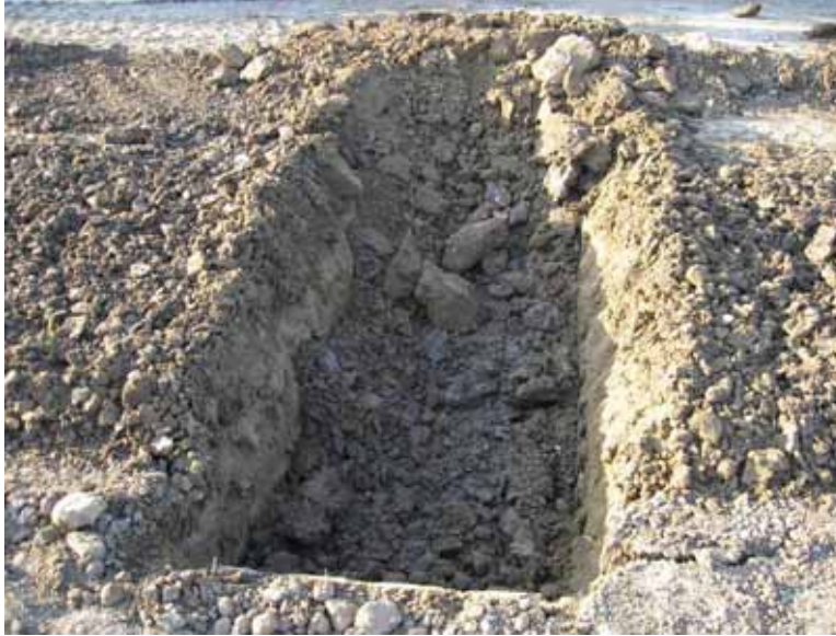
Figure 153. Excavated trench for roller identification of a soft spot
