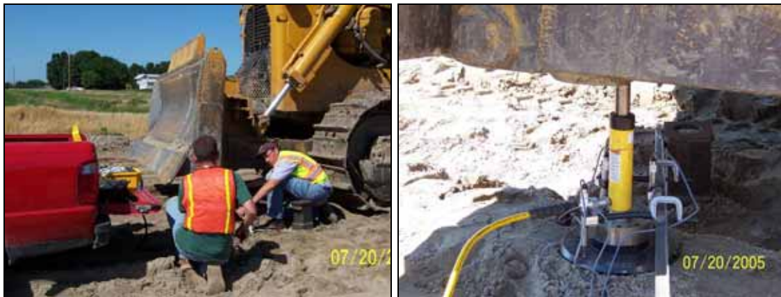
Figure 179. Plate load test setup and performance
