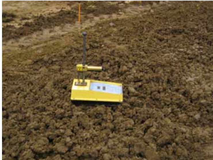
Figure 4. Moisture and density determination using nuclear moisture-density gauge for 0 roller passes
