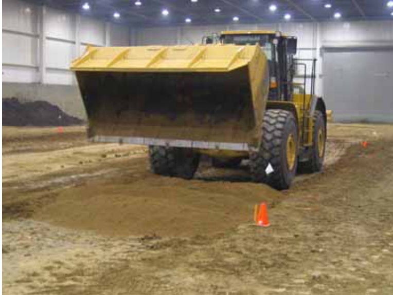
Figure 2. Placement of soil in excavated and stabilized test strip pit
