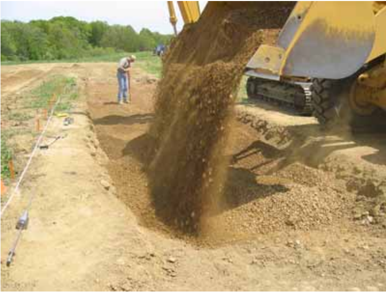
Figure 148. Placement of fill in test strip
