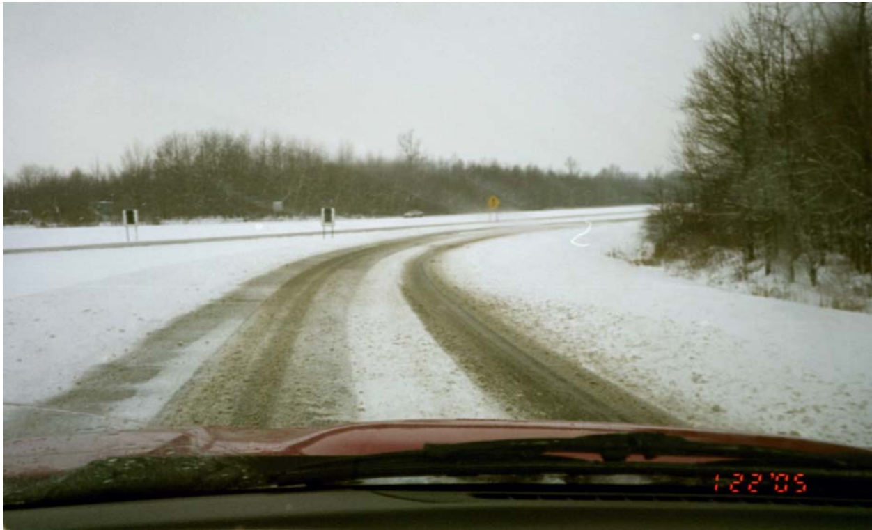
Figure 89: Picture documenting typical road condition on the free way entrance ramp near I-76 westbound after 11.30 am on January 22, 2005.
