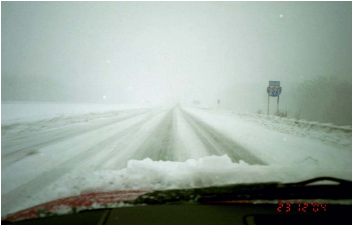
Figure 20: Picture documenting typical road condition taken on main line of I-271 on December 23, 2004. The road is covered with snow, ice, and slush.
