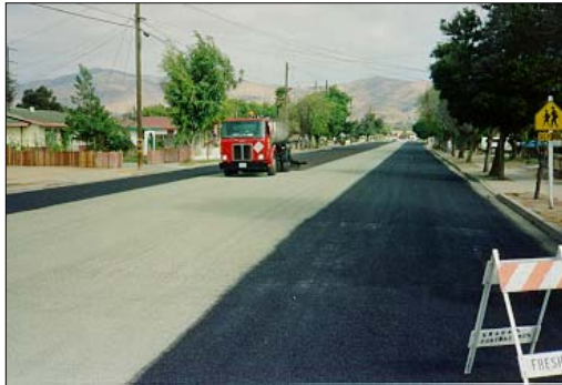
Figure 2: Fog Seal Application
