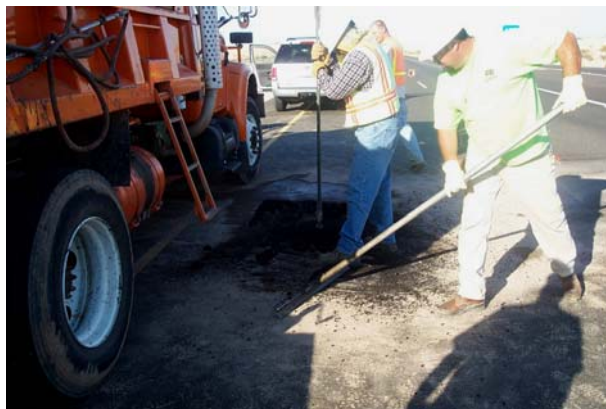
Figure 6: Throw and Roll Patching
