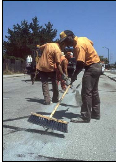
Figure 22: Brooming Blotter Coat Over a Treated Crack
