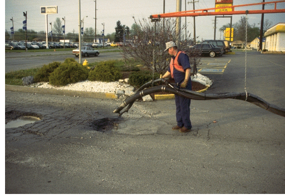
Figure 13: Application of Tack Coat
