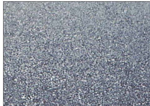
Figure 5: Suitable Surface, Open Graded HMA
