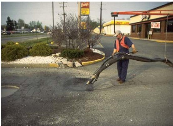
Figure 14: Filling the Prepared Hole
