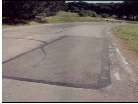
Figure 16: Edge Seal Application
