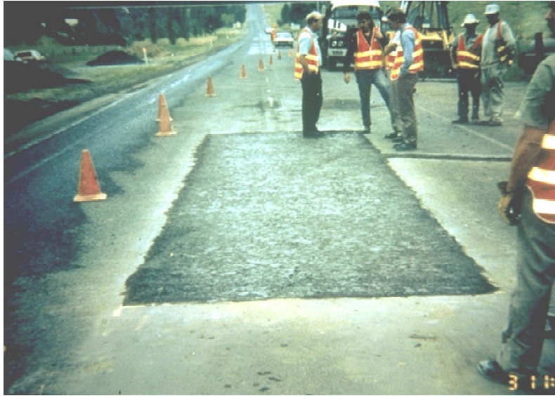
Figure 17: Dig Out Project
