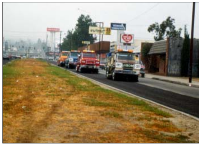
b) Spreading of Aggregate
