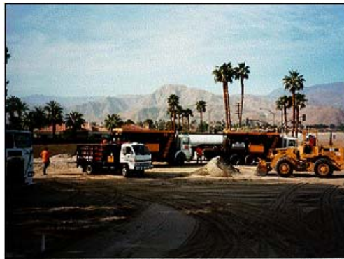
Figure 9: A Typical Stockpile and Project Staging Area
