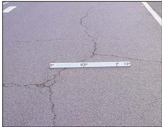
Figure 4: Block Cracking
