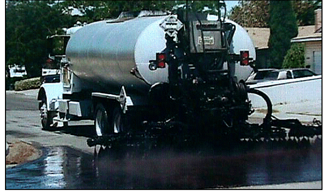
Figure 8: Spray Distributor
