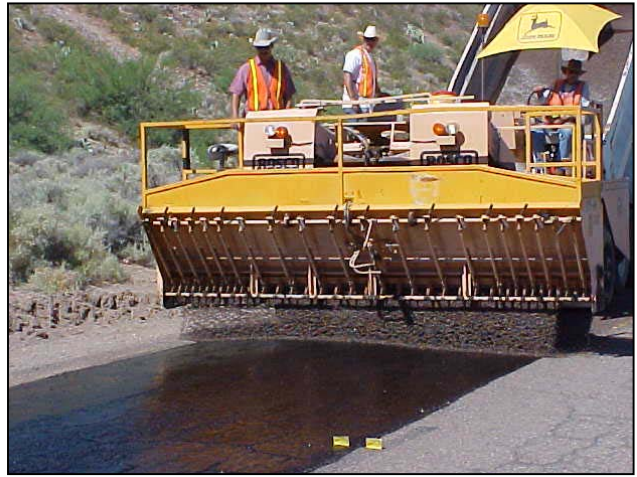
b) Spreading of Aggregate
