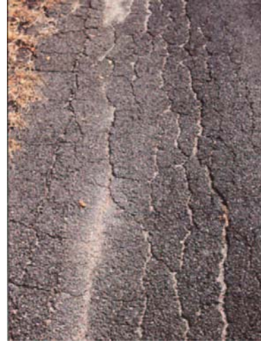
Figure 6: Edge Cracking
