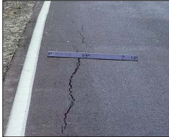
Figure 2: Longitudinal Cracking
