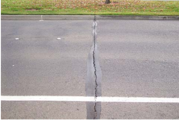
Figure 5: Reflection Cracking
