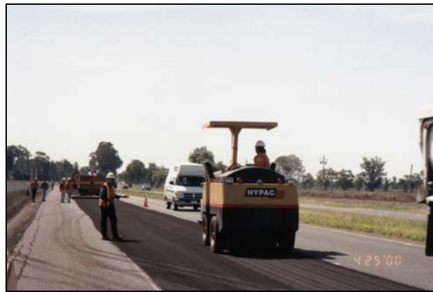
Figure 13: Pneumatic (Rubber Tired) Roller
