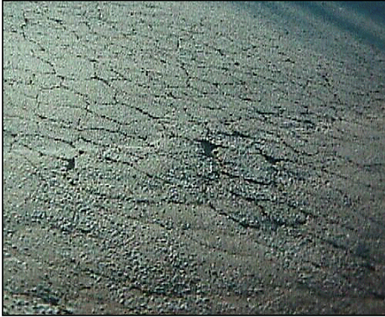
Figure 1: Fatigue Cracking
