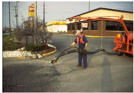
Figure 15: Application of Finish Coat
