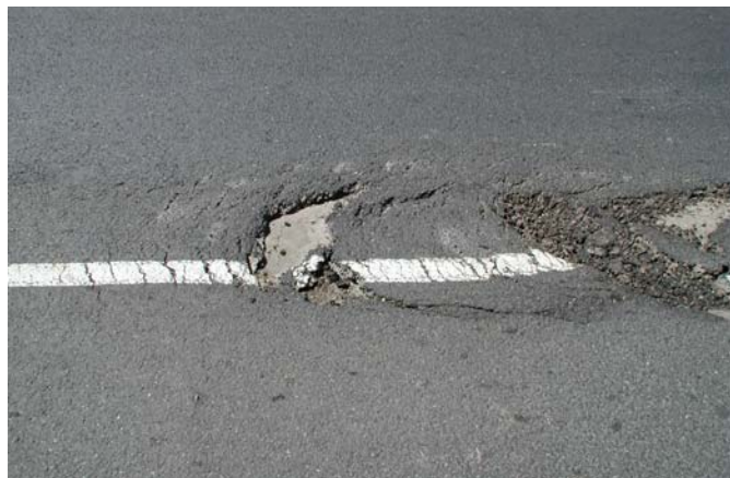
Figure 7: Slippage Cracking
