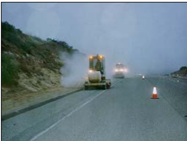
Figure 14: Brooming Process, Shown on a Shoulder Seal
