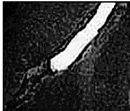
Figure 19: Backer Rod Installed Into Crack Channel
