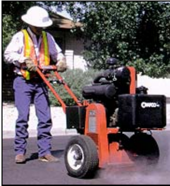
Figure 17: Crack Routing Operation
