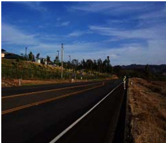
a) High Quality Longitudinal Joint
