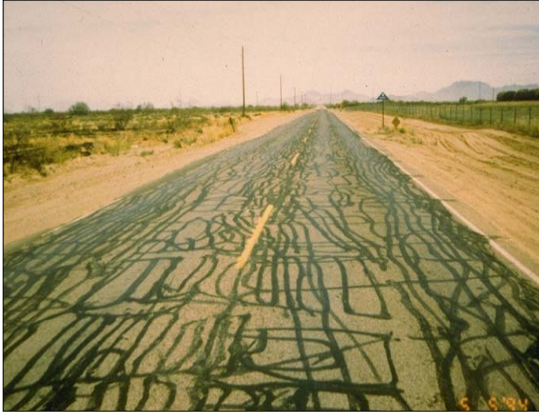
Figure 23: Excessive Sealant
