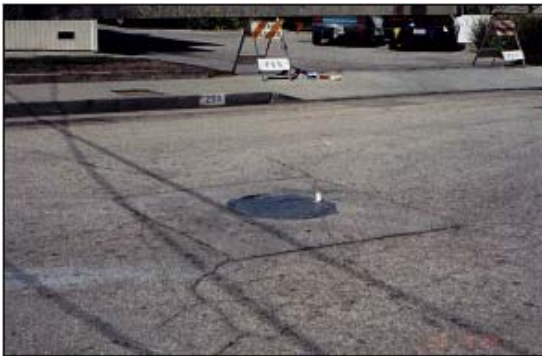
c) Cover Utilities with Kraft Paper
