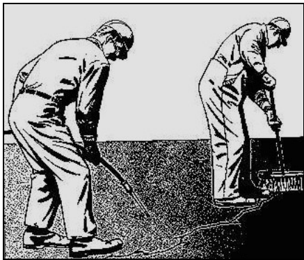
Figure 18: Manual Crack Cleaning
