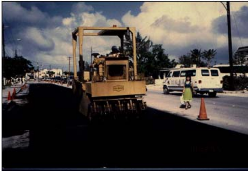
Figure 19: Rolling a Slurry Surfacing
