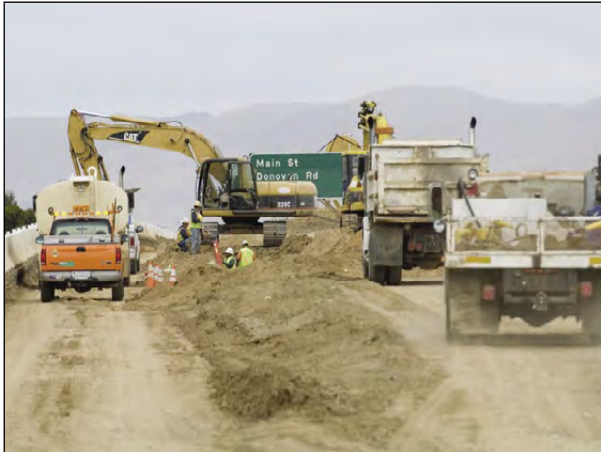
Caltrans widens Highway 101 near Santa Maria.
