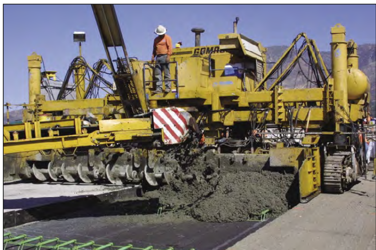
Placement of new concrete pavement with dowel bars
