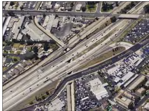
The I-5 Gateway Project area before work began
