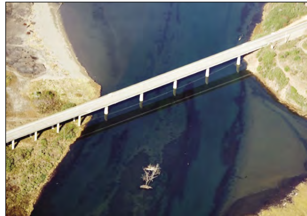
Ten mile River Bridge, north of Fort Bragg
