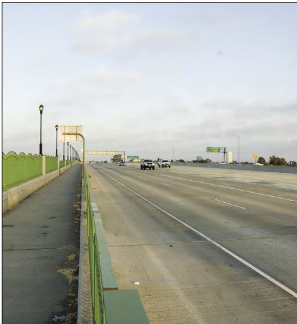
New Santa Clara River Bridge in Ventura County
