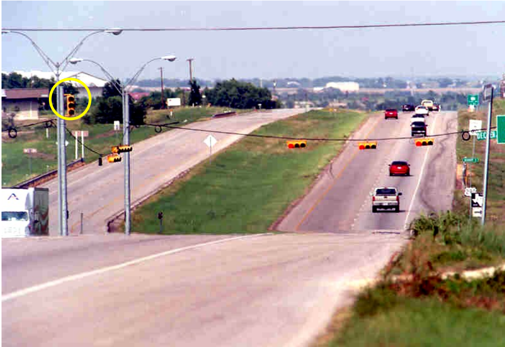
(B) Traffic Signal More Visible Beyond Crest. Figure 8-1. Traffic Signal Just Visible Beyond Crest of Hill.
