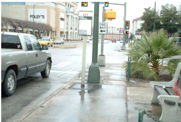
Figure 7-13. Poles and Signs in Sidewalk on Southeast Corner of Intersection Looking North.
