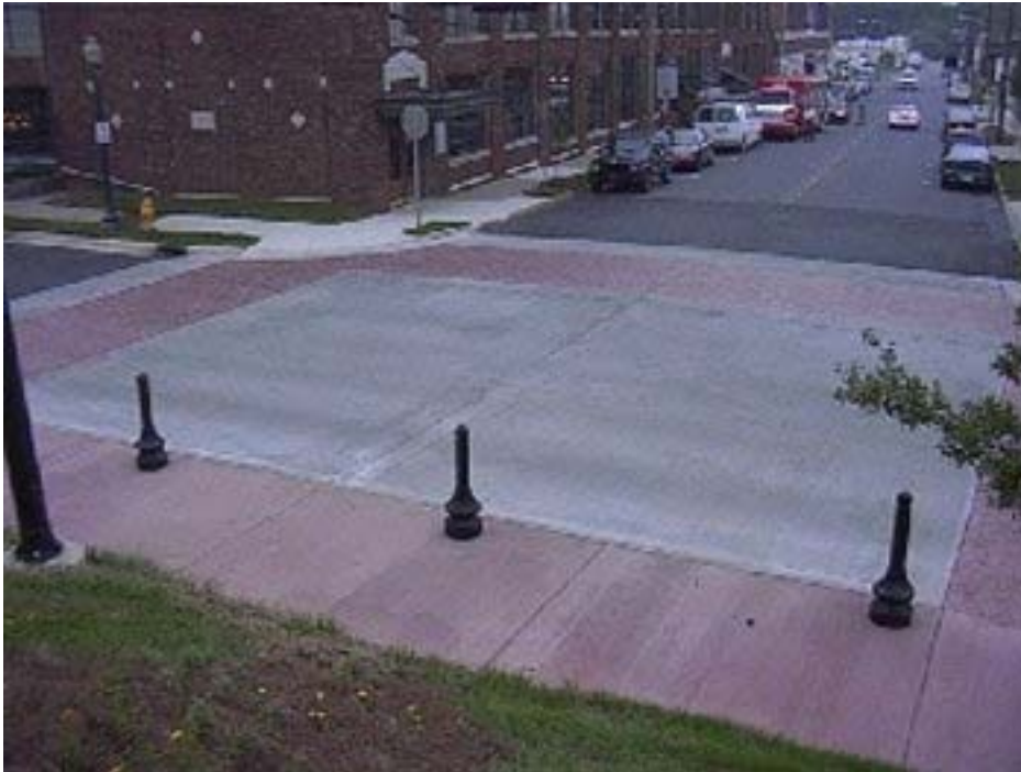
Figure 7-32. Raised Intersection in Portland. 9
