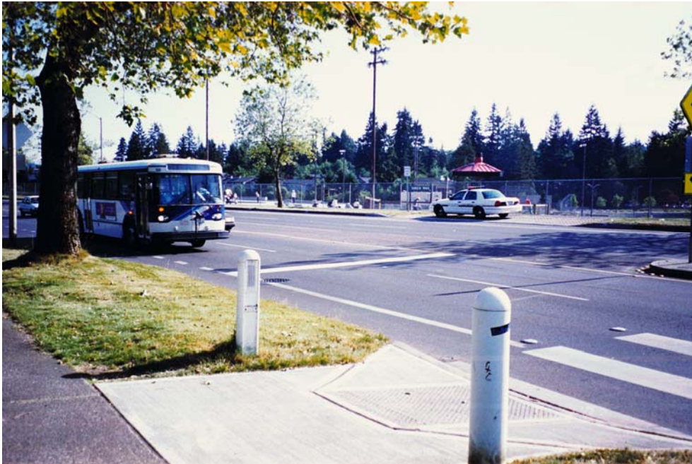
Figure 7-30. Example of Bollard Detection System.
