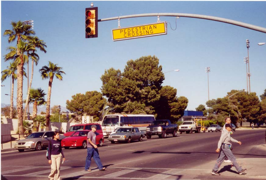
Figure 7-41. Example of Pedestrian Crossing Sign on Mast Arm in Tucson, Arizona.
