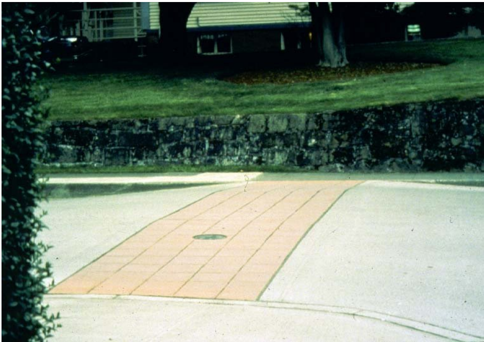
Figure 7-31. Example of Raised Crosswalk in Portland, Oregon. 9
