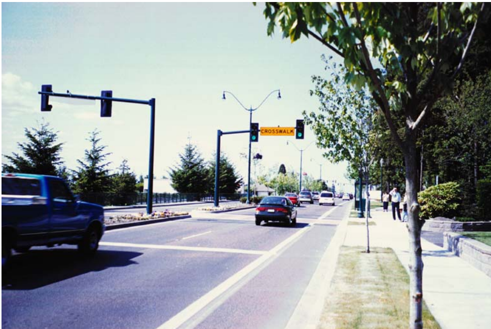
Figure 7-33. Example of a Midblock Signal in Washington.
