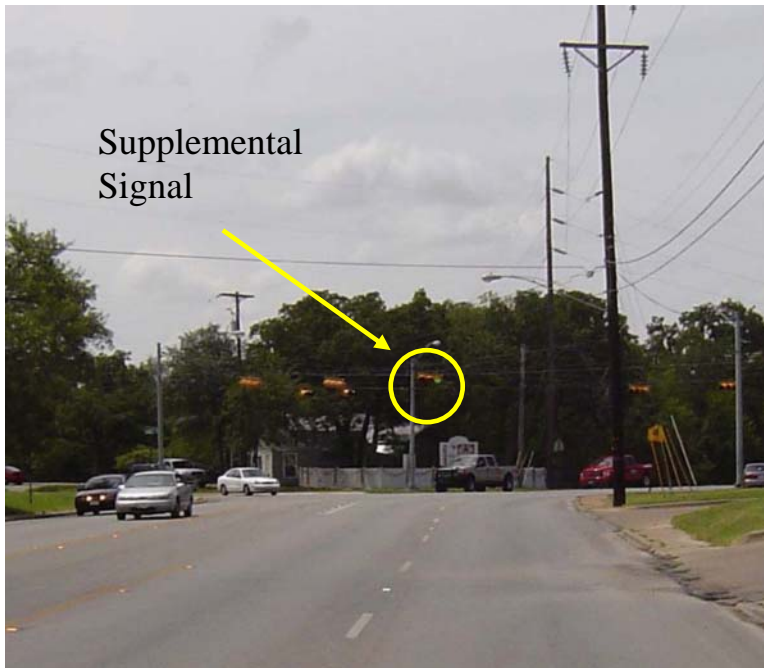
Figure 8-2. Supplemental Signal Due to Horizontal Curve at Villa Maria and Cavitt Ave.
