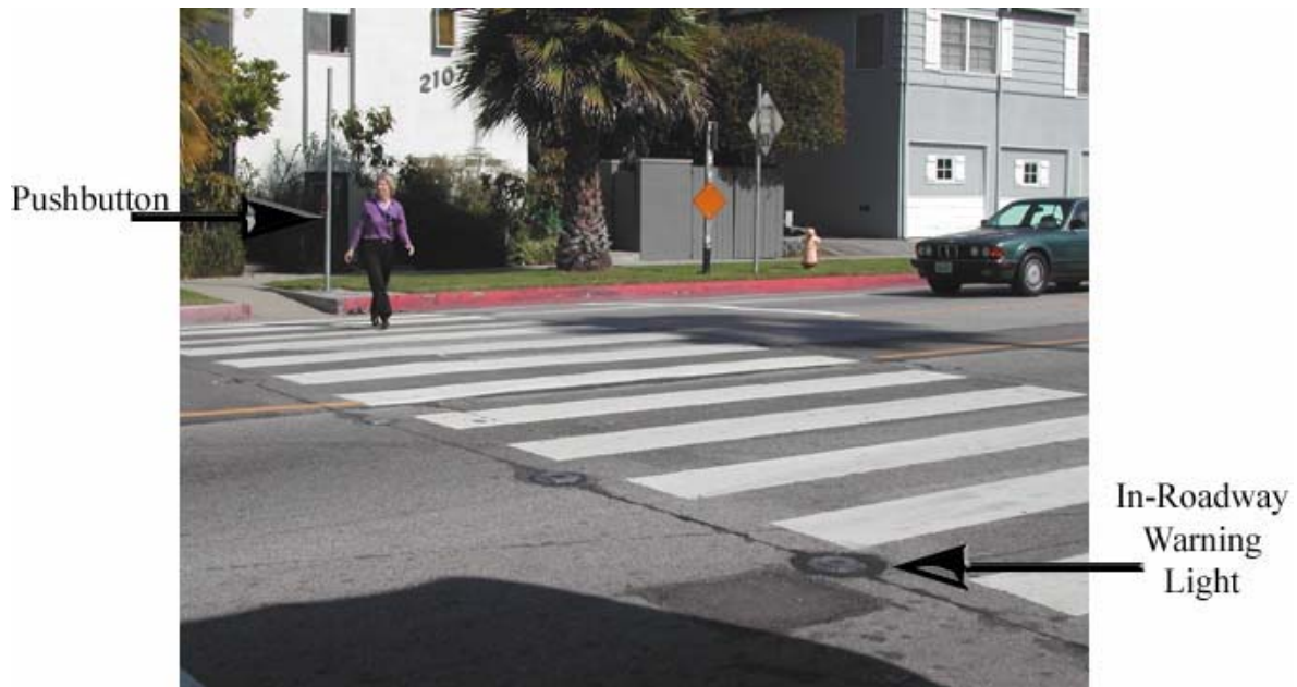
Figure 7-28. Example of In-Roadway Warning Lights.
