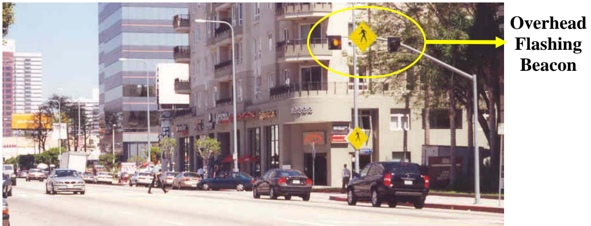
Figure 7-29. Example of Overhead Flashing Beacon.
