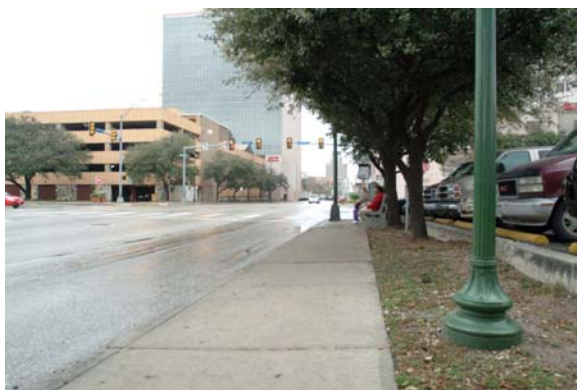
Figure 7-12. Cross-Slope on Approach in Sidewalk on Northeast Corner of Intersection Looking West.
