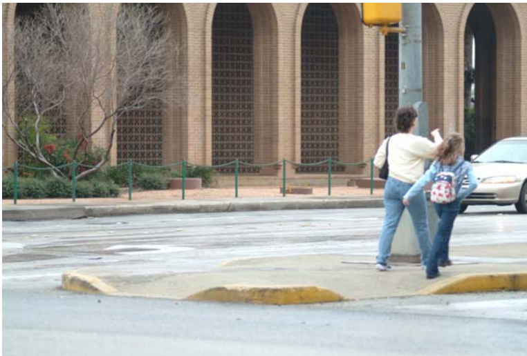
Figure 7-6. Uneven Island and Ramp with No Crosswalk (on Southwest Corner of Intersection).
