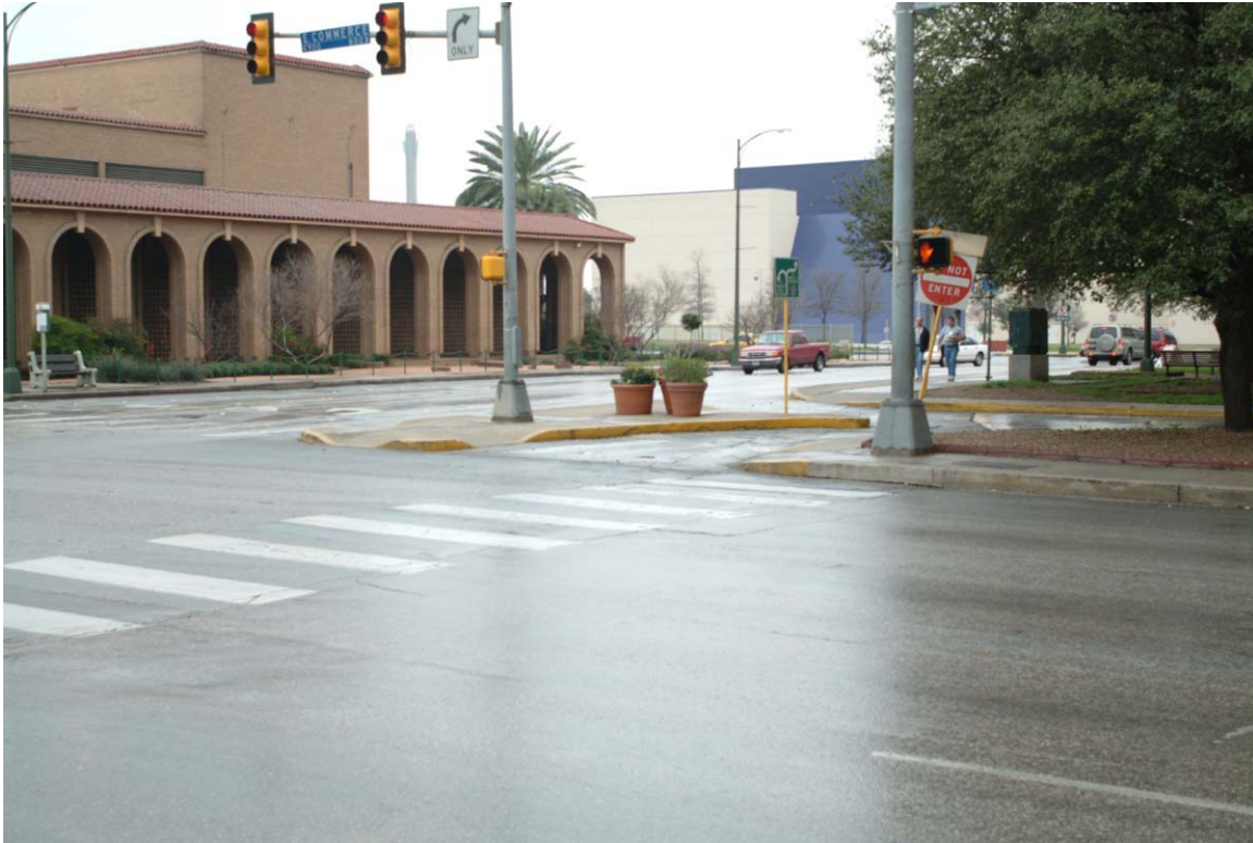
Figure 7-5. View of Exits from Parking Garage and Corner Island (Southwest Corner of Intersection).
