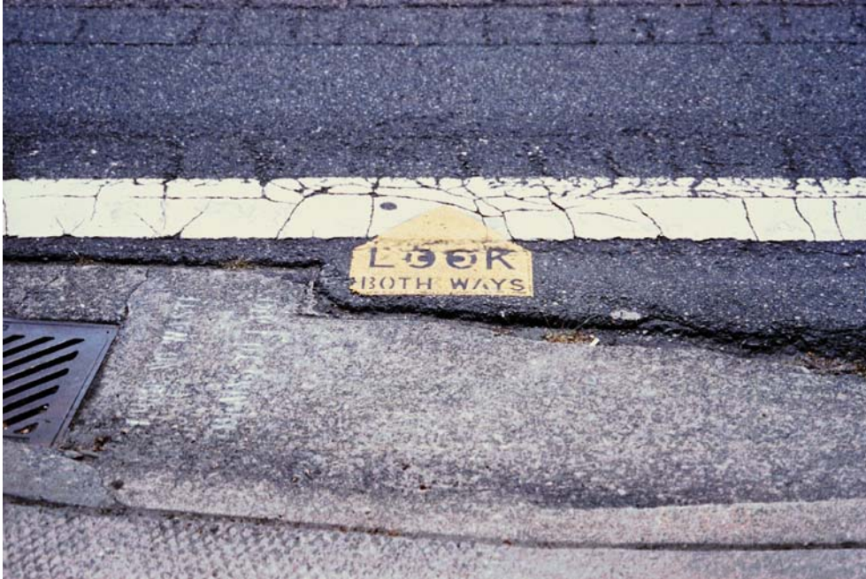
Figure 7-22. Look Both Ways Pavement Markings.
