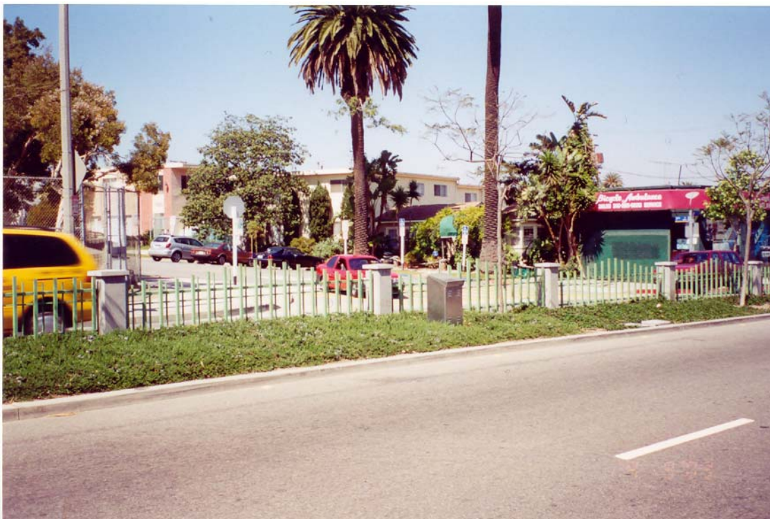
Figure 7-27. Example of a Pedestrian Railing in a Median in Santa Monica, California.
