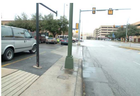
Figure 7-11. Light Pole in Narrow Sidewalk on Northeast Corner of Intersection Looking South.
