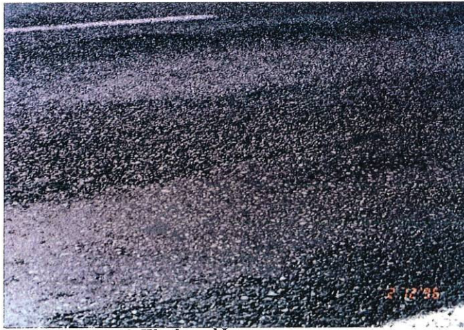
Photo 4, MP 208.09, Westbound Lanes Wheelpaths in the truck lane where the MCD has turned fat.
