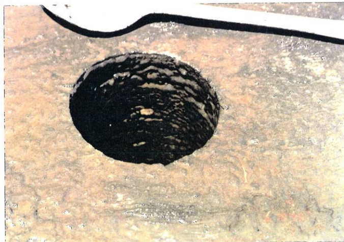
Photo 8, MP 202.49, Westbound Truck Lane Stripped Asphalt Class B beneath the MCD surface in the left wheelpath. The MCD surface appears fat and the core appears very dense.
