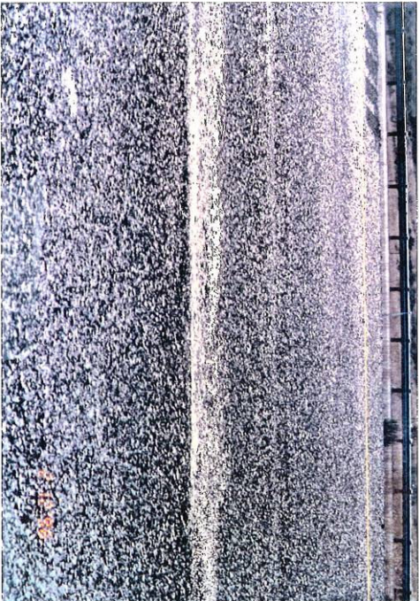
Photo 16, MP 208.84, Westbound Truck Lane Water "dammed" by compressed MCD on the high side of the wheel rut.
