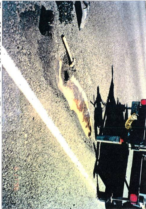
Photo 22, MP 195.68, Eastbound Truck Lane Isolated pothole. Stripping occurs almost full thickness
