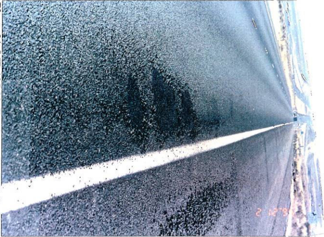
Photo 22, MP 195.68, Eastbound Truck Lane Isolated pothole. Stripping occurs almost full thickness
