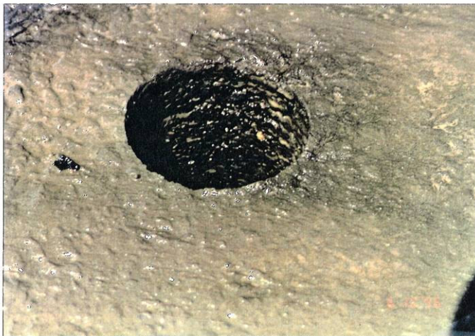
Photo 10, MP 206.69, Westbound Truck Lane Stripped Asphalt Class B beneath the MCD surface in the left wheelpath. The MCD surface appears fat and the core appears very dense.
