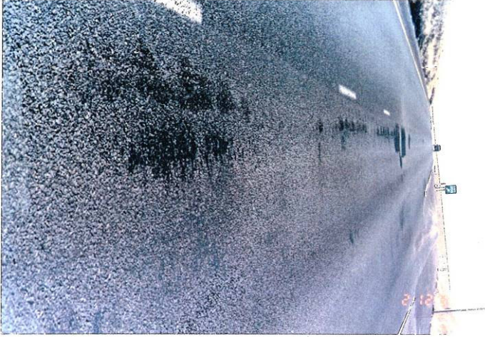
Photo 16, MP 208.84, Westbound Truck Lane Water "dammed" by compressed MCD on the high side of the wheel rut.
