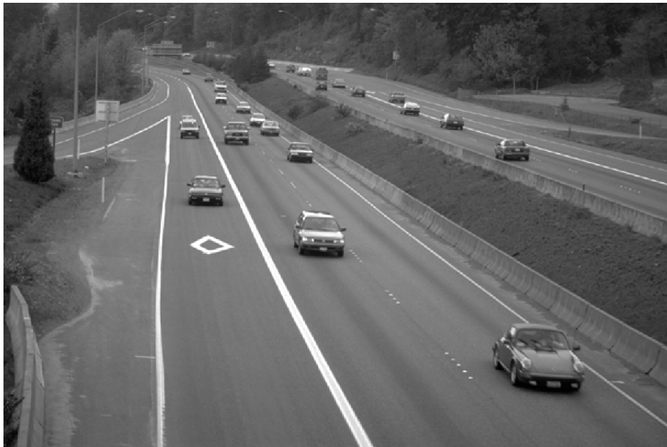
Figure 6-35. I-405, Seattle Concurrent Flow HOV Lanes (Shoulder Location). (10)
