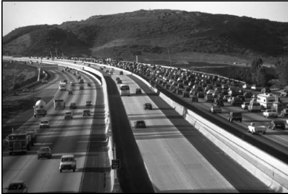
Figure 6-1. HOV Lane in San Diego, CA.
