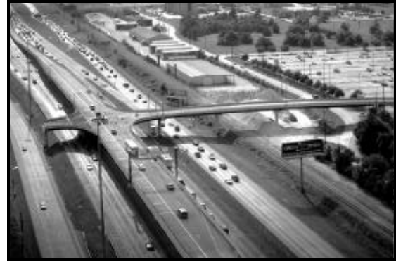
Figure 6-15. Grade Separated Interchange. (9)
