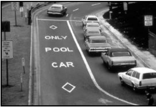
Figure 6-20. Two-Lane Entrance Ramp with HOV Bypass. (9)
