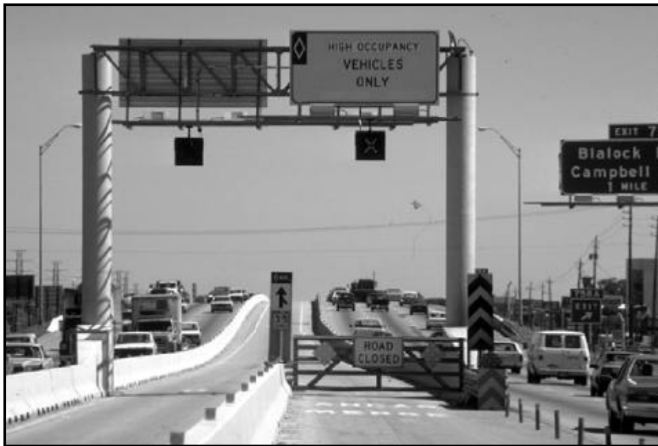
Figure 6-29. Houston HOV Slip Ramp. (9)
