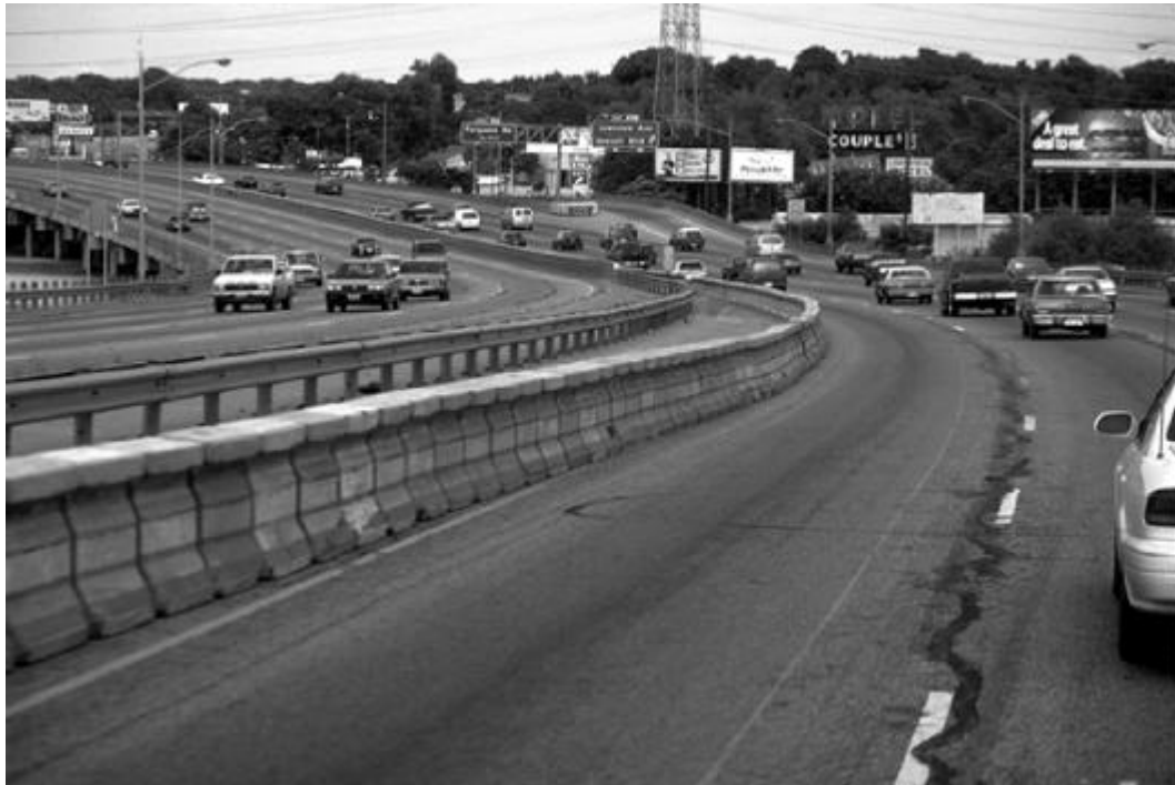
Figure 6-23. Movable Barrier. (9)
