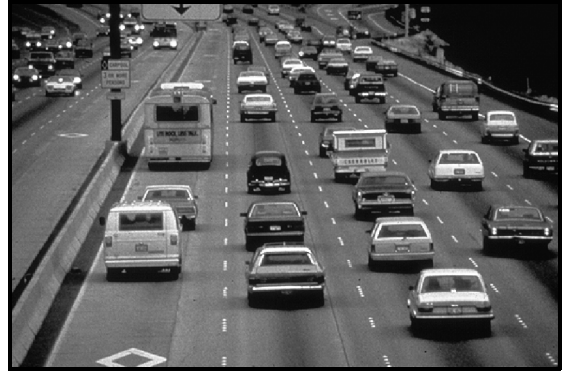
Figure 6-34. I-5, Seattle Concurrent Flow HOV Lanes (Median Location). (9)
