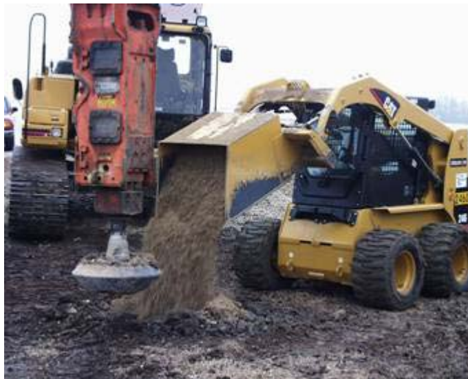
Figure 5.5. High-energy, low-frequency hammer used for the construction of Geopier foundations [photo courtesy of the Iowa DOT].
