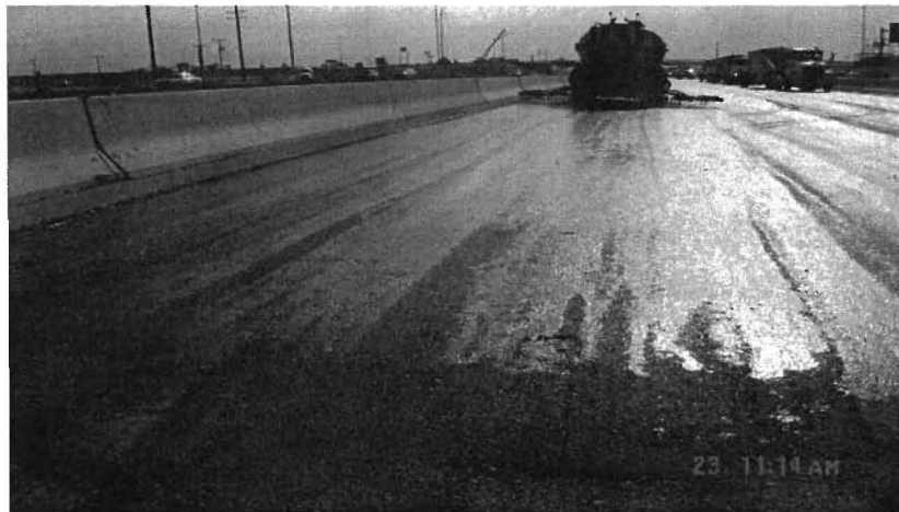
Figure 7.11 - Tack Coat Application at Joe Battle (I-10 Eastbound)
