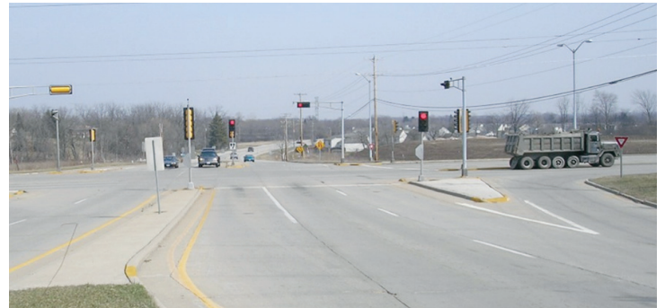
Raised channelization medians better delineate intersection approaches, and retroreflective markings make curbs and lanes more conspicuous.
