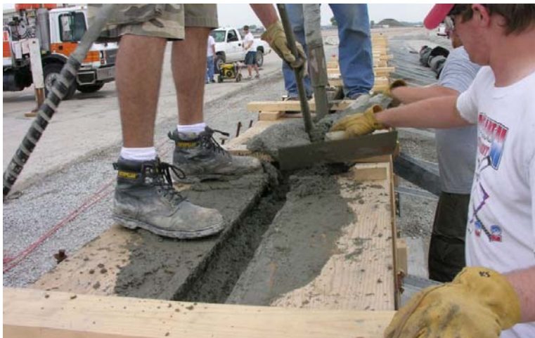
Figure 58. TL-5 Median Barrier Construction
