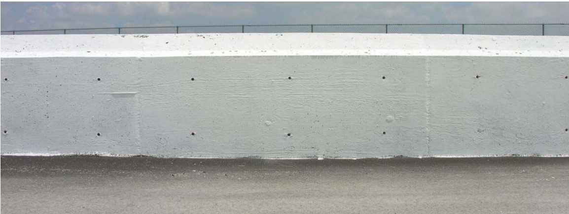
Figure 60. TL-5 Concrete Median Barrier
