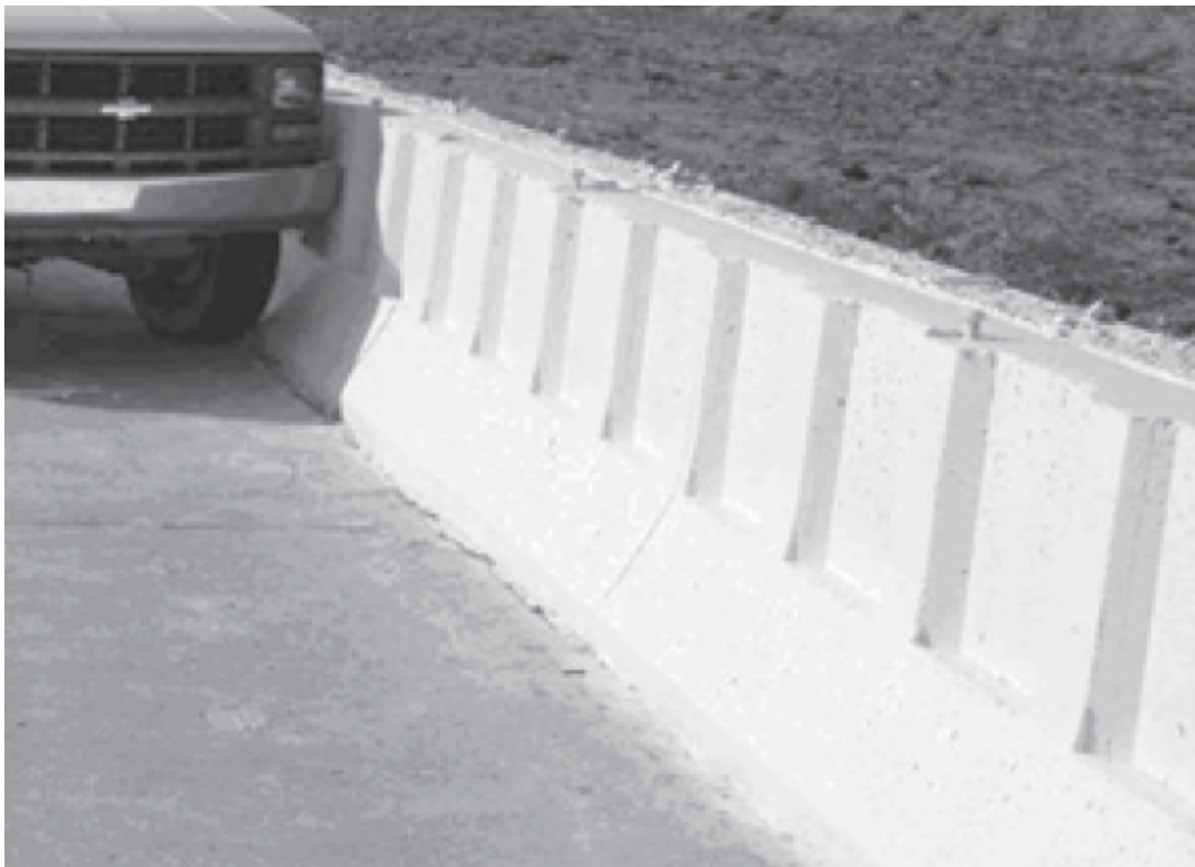
Figure 38. Examples of Texturing [38] and Vertical Asperities [79]
