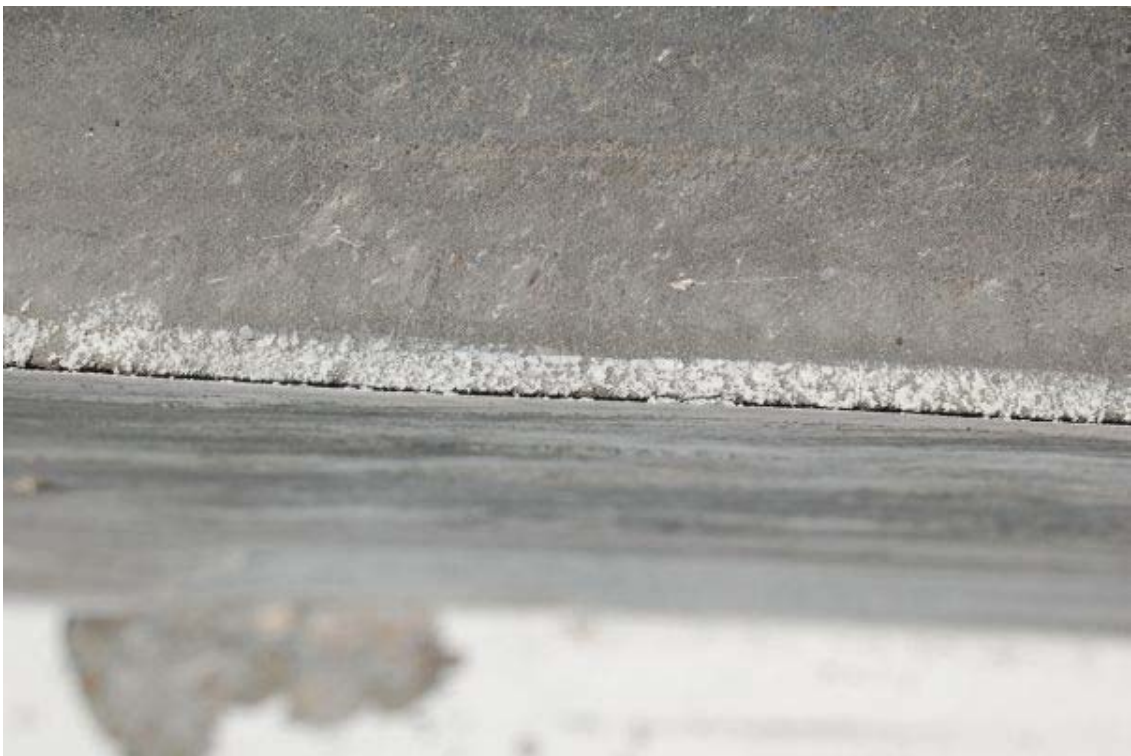
Figure 84. Front-Side Barrier Asphalt Gaps Near Impact, Test TL5CMB-2
