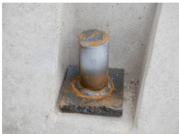
Barrier No. 4 Non-Traffic Side Downstream
