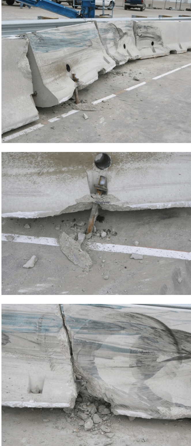
Figure 63. System Damage, Test No. TCBT-2
