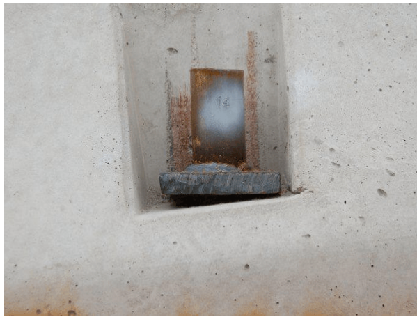
Barrier No. 3 Traffic Side Upstream
