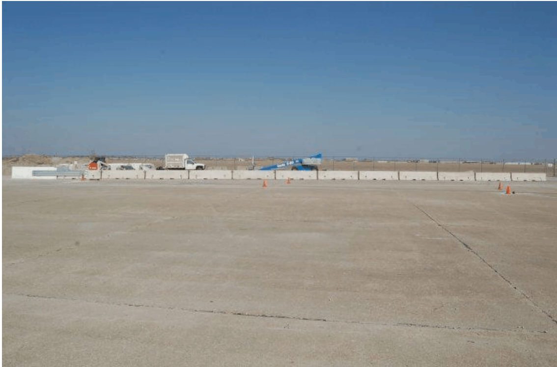
Figure 21. Temporary Concrete Barrier to Permanent Concrete Barrier Transition, Test No. TCBT-1 and TCBT-2
