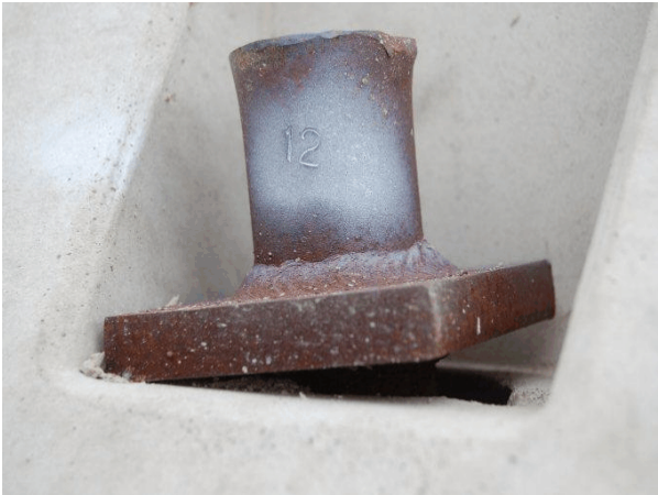
Barrier No. 2 Non-Traffic Side Upstream
