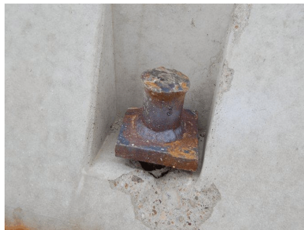
Barrier No. 1 Traffic Side Upstream
