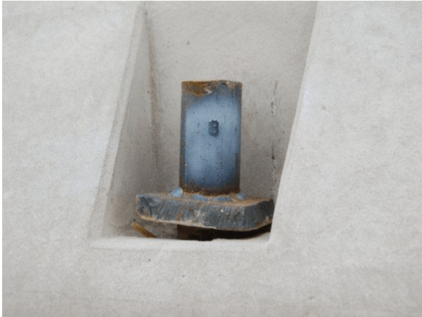
Barrier No. 2 Traffic Side Midspan
