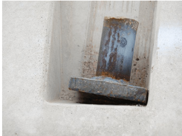
Barrier No. 2 Traffic Side Upstream
