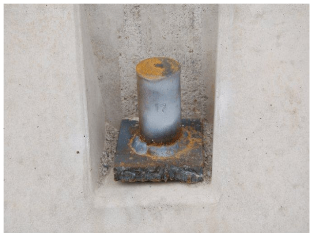
Barrier No. 4 Traffic Side Downstream
