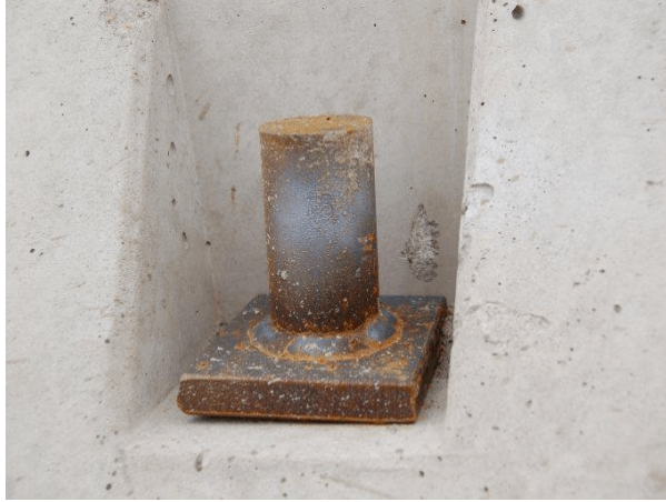
Barrier No. 3 Traffic Side Downstream
