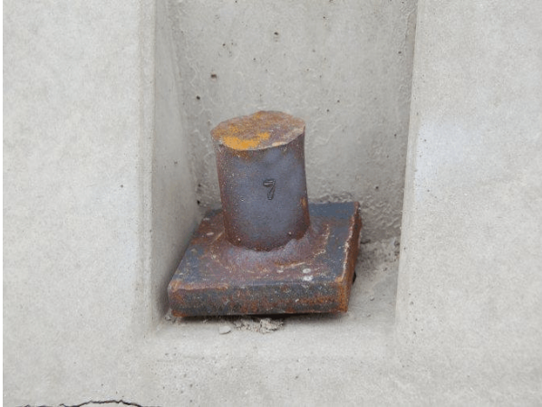
Barrier No. 2 Traffic Side Downstream
