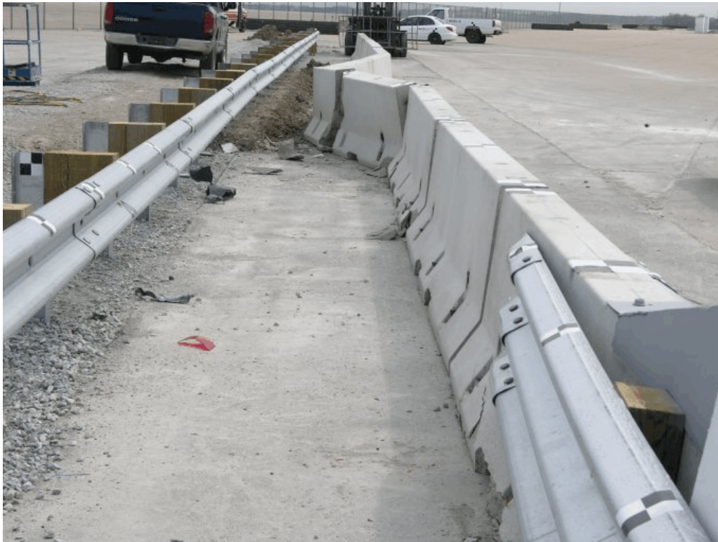
Figure 62. System Damage, Test No. TCBT-2
