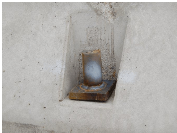
Barrier No. 3 Non-Traffic Side Downstream
