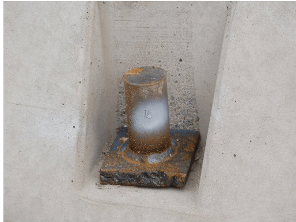
Barrier No. 3 Non-Traffic Side Upstream
