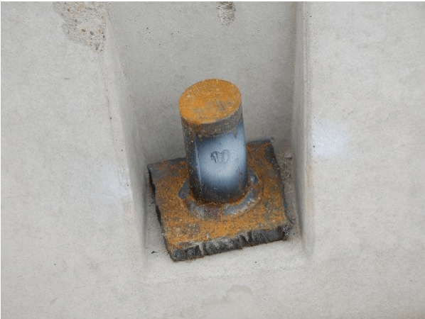
Barrier No. 2 Non-Traffic Side Downstream
