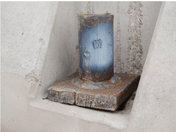
Barrier No. 2 Non-Traffic Side Midspan
