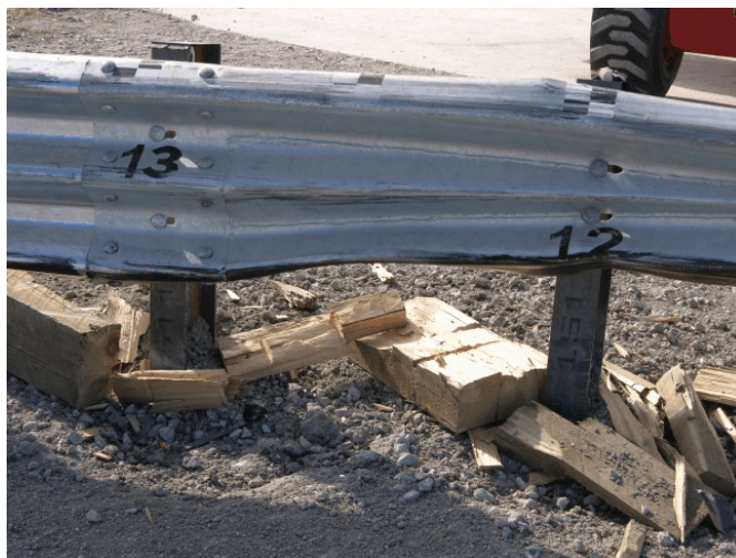
Figure 110. Post Nos. 10 through 13 Damage, Test MWT-5
