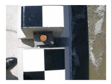
Figure 9. Barrier Connection Joints
