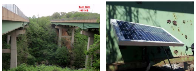
I-95 Bridge site and the solar-wind Hybrid power
