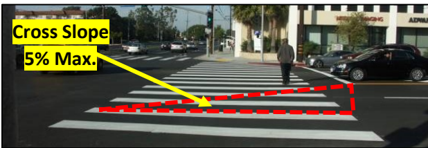
Figure 71: Pedestrian Street Crossing without Yield or Stop Control
