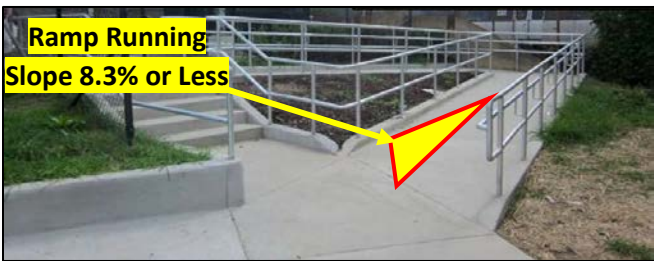
Figure 104: Ramp Running Slope
