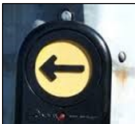
Figure 83: Tactile Arrow Visual Contrast with Pushbutton
