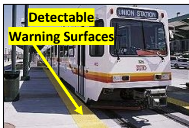
Figure 59: DWS at Boarding and Alighting Areas
