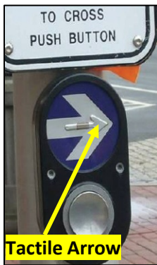
Figure 82: Vibro-Tactile Walk Indicators
