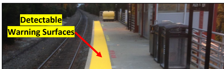
Figure 58: DWS at Boarding Platforms
