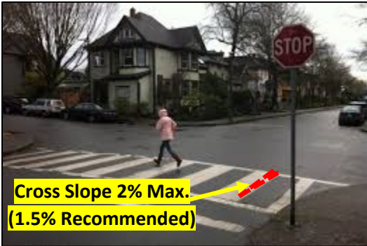
Figure 12: Pedestrian Street Crossing with Stop Control
