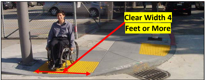
Figure 32: Curb Ramp Width
