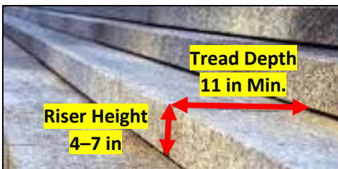
Figure 110: Riser and Tread Dimensions
