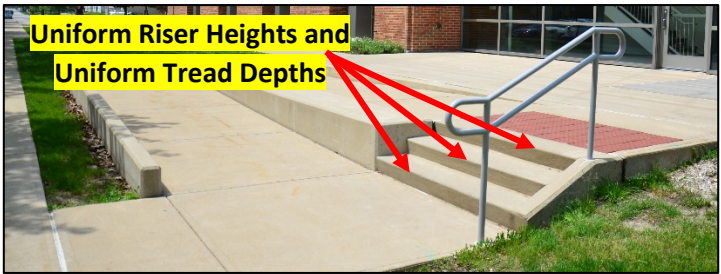
Figure 109: Uniform Riser Height and Tread Depth
