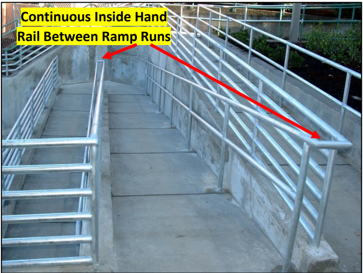
Figure 113: Handrail Continuity Requirement
