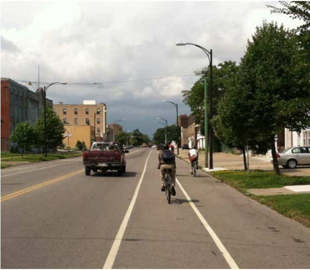
Bike Lane on Fillmore Ave
