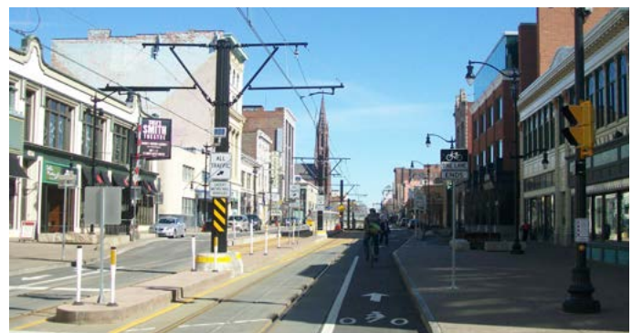
Main Street was recently reopened to vehicles.
