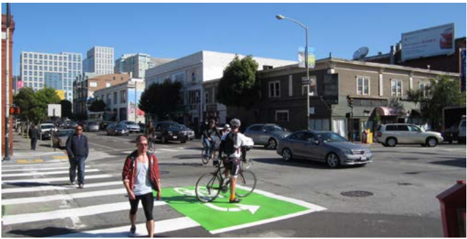
Two-stage turn queue boxes provide a holding area for bicyclists to queue, allowing them to cross an intersection in two stages in the San Francisco area. This crossing pattern is more comfortable, especially for less experienced bicyclists.
