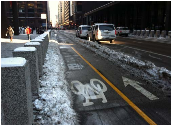
Chicago, IL: Small plows/bob-cats clear cycle tracks that are separated from the roadway by bollards. Alternatively, delineator posts can be removed during winter and larger plows clear cycle track and painted buffer areas to the curb
