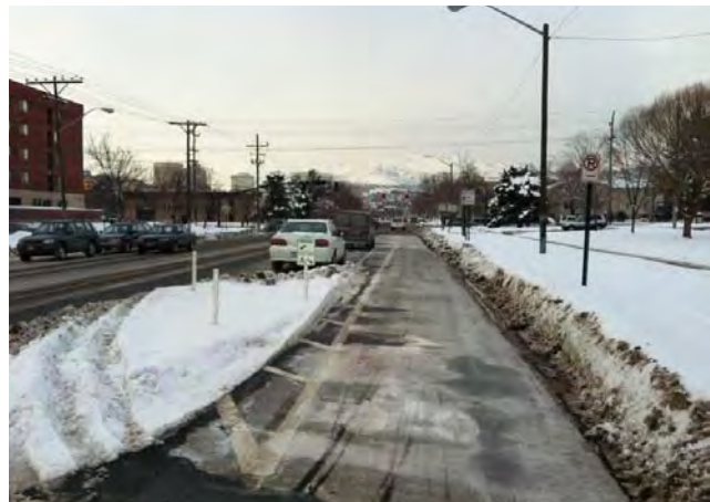
Above: Protected cycletrack in Salt Lake City, UT after small truck plow snow removal. Photo Credit: Travis Jensen
