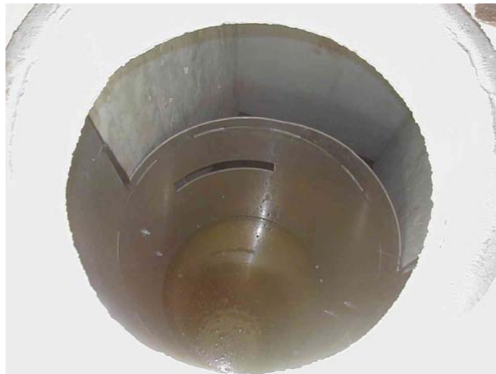
Figure 21. Cleanout of the settling chamber for the hydrodynamic settling device.
