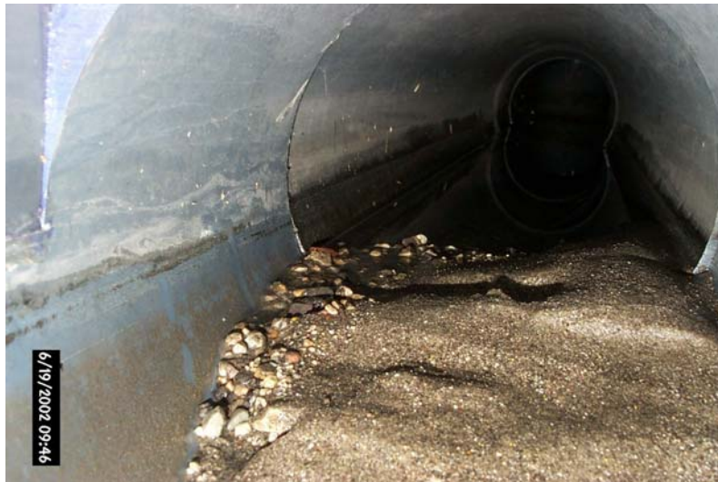
Figure 22. Cleanout of the 8 in. inlet pipe for the hydrodynamic settling device.
