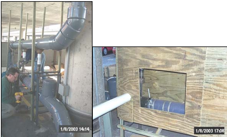
Figure 7. Piping modification of the hydrodynamic settling device.
