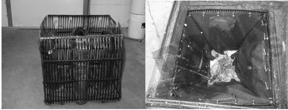
Figure 6. DrainPac catchbasin insert.
