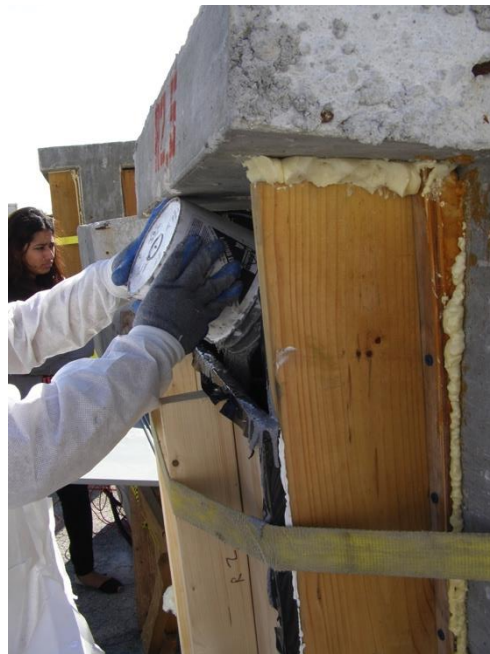
Figure 4-6: Mixing and casting of epoxy pourback
