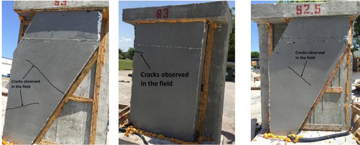
Figure 5-4: Cracks in pourback specimens
