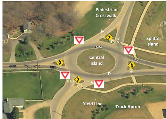
Tienken Road and Runyon Road/Washington Road Rochester Hills, MI
