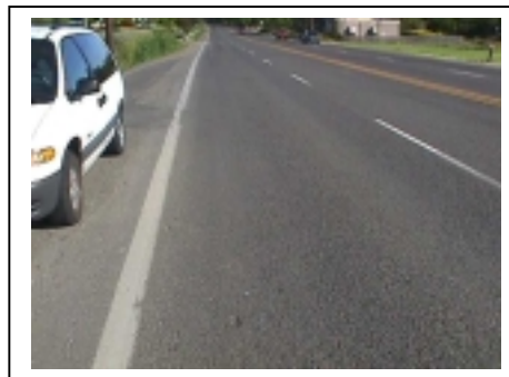
#31 Looking back north @ 12.9 SB
