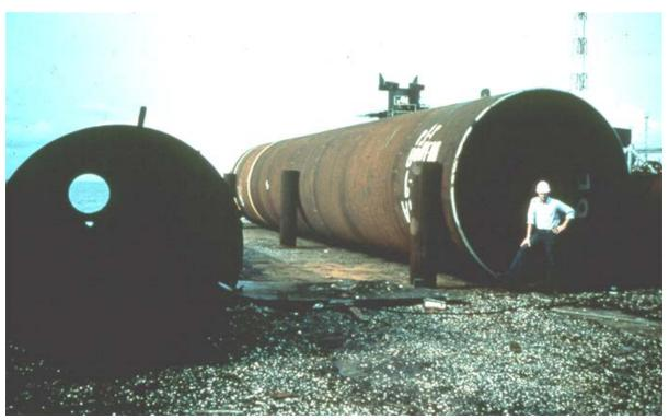
Figure 6-13 Large diameter open end pipe piles.
