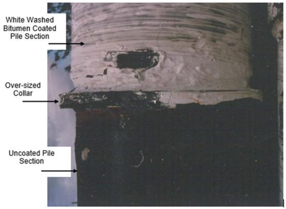
Figure 7-62 Over-sized collar for bitumen coating protection.
