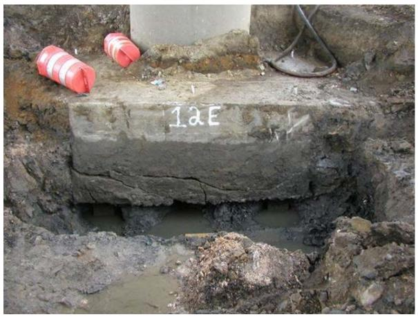
Figure 3-15 Cracked pile cap from lateral soil movements (courtesy DelDOT).
