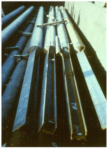
Figure 6-25 Steel pipe - H-pile composite piles.
