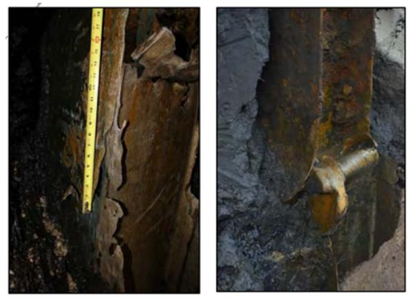
Figure 3-10 Corrosion and resulting buckling of foundation pile (courtesy Wisconsin Department of Transportation).
