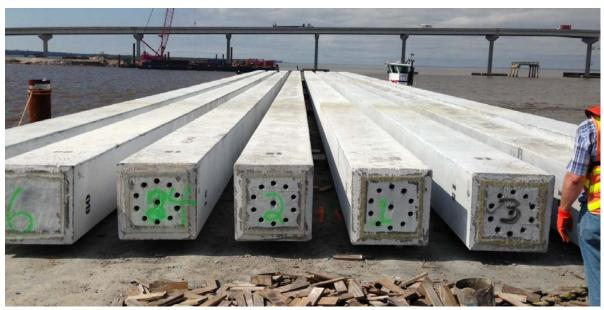
Figure 6-21 Square prestressed concrete piles.
