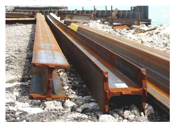
Figure 6-10 H-piles with driving shoes.
