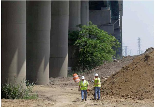
Figure 3-14 Tilting columns adjacent to stockpile (courtesy DelDOT).
