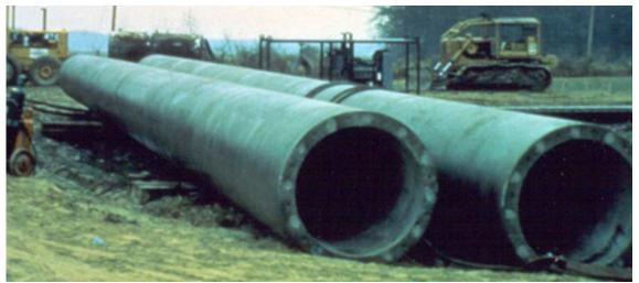
Figure 6-23 Concrete cylinder pile.
