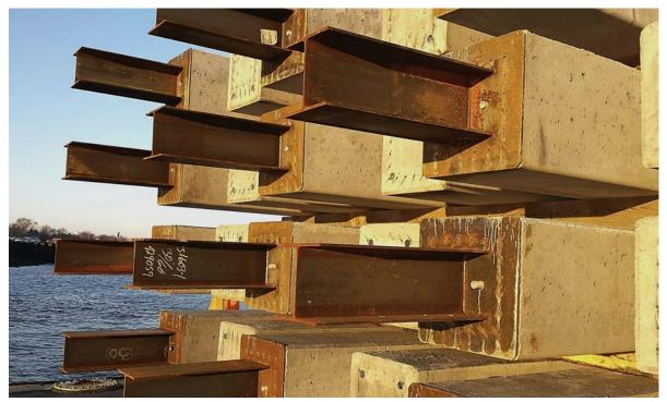
Figure 6-24 Precast concrete piles each with H-pile stinger.
