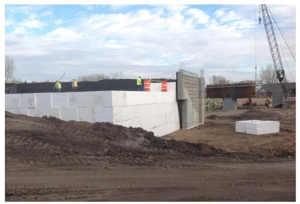
Figure 7-61 Geofoam block approach embankment (courtesy MnDOT).
