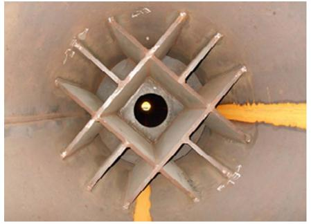
Figure 6-15 Constrictor plate installed inside pipe pile.
