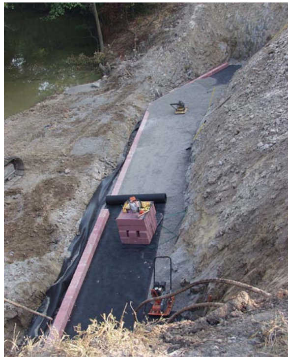
Figure 51. Reinforcement rolled out parallel to wall face.
