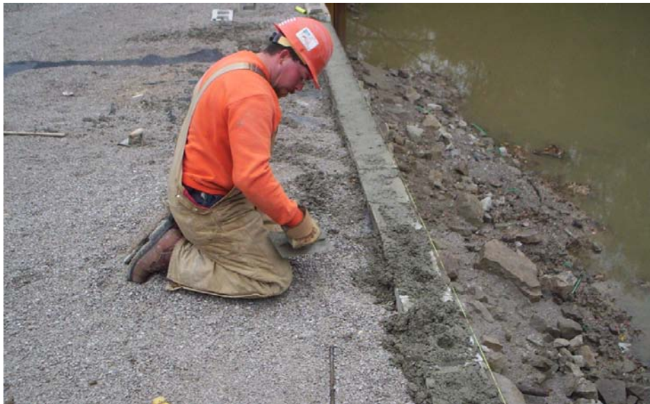
Figure 60. Photo. Connecting the top courses of blocks.
