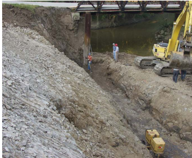
Figure 47. Photo. RSF cut preparation.
