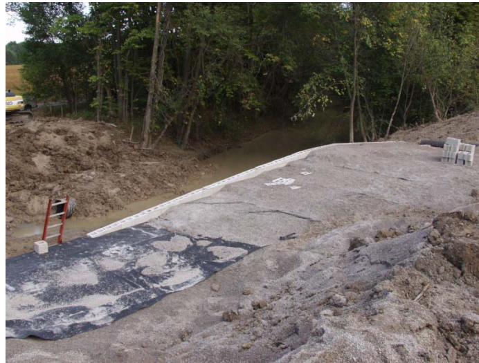
Figure 53. Photo. Superelevation reinforcement layers.
