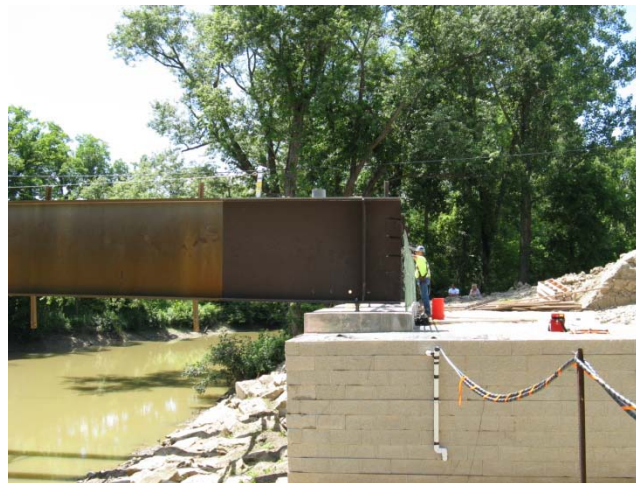
Figure 71. Photo. Steel girder on CIP footing.
