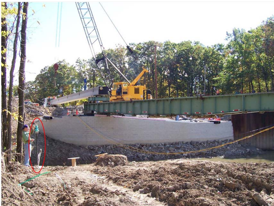
Figure 39. Photo. Location of total station reference pole.
