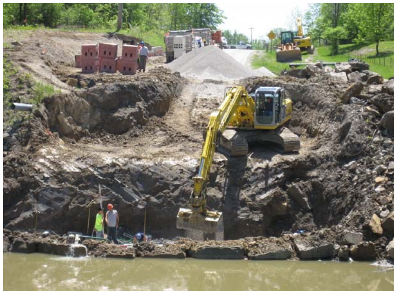
Figure 46. Photo. RSF excavation below stream level.
