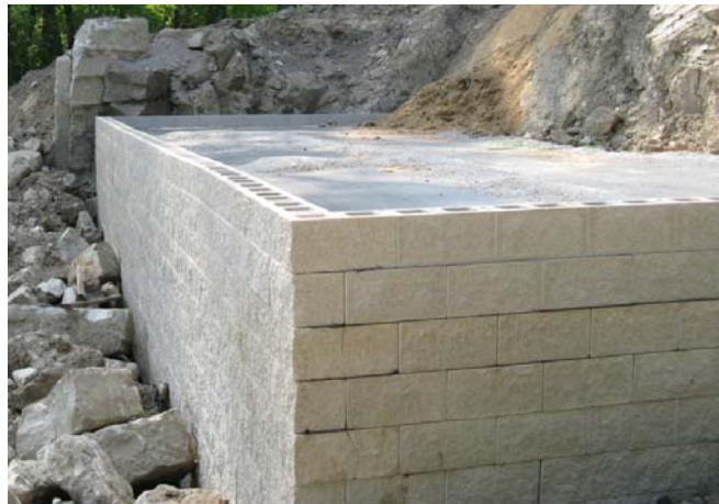
Figure 57. Photo. Right-angle wall corner.
