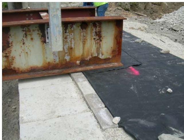
Figure 73. Photo. Additional reinforcement under beam.
