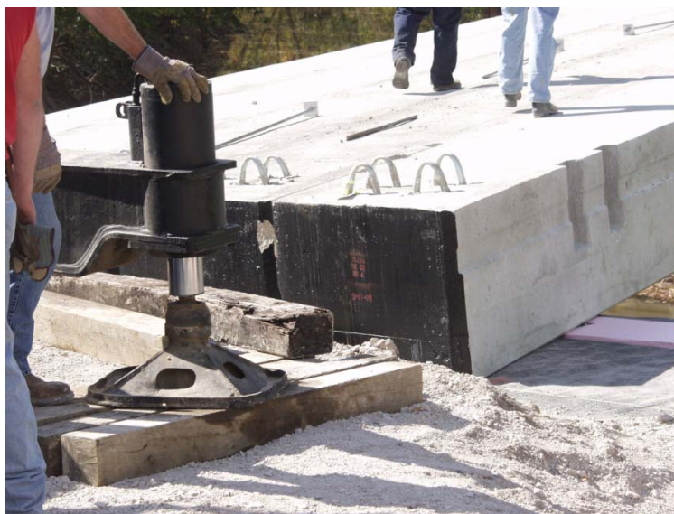
Figure 8. Photo. Bitumen coating on concrete beam ends.
