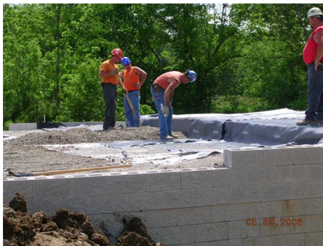
Figure 77. Photo. First 6-inch fill lift.
