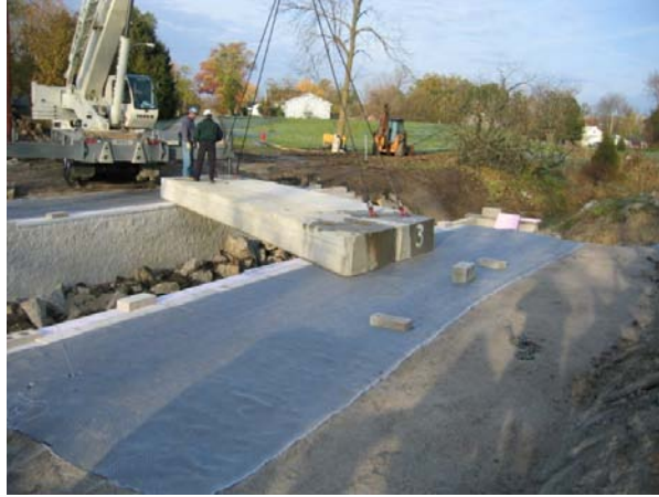
Figure 63. Photo. Box beam placed on beam seat.
