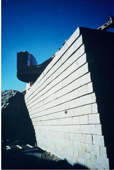
Figure 55. Photo. Negative batter wall face.
