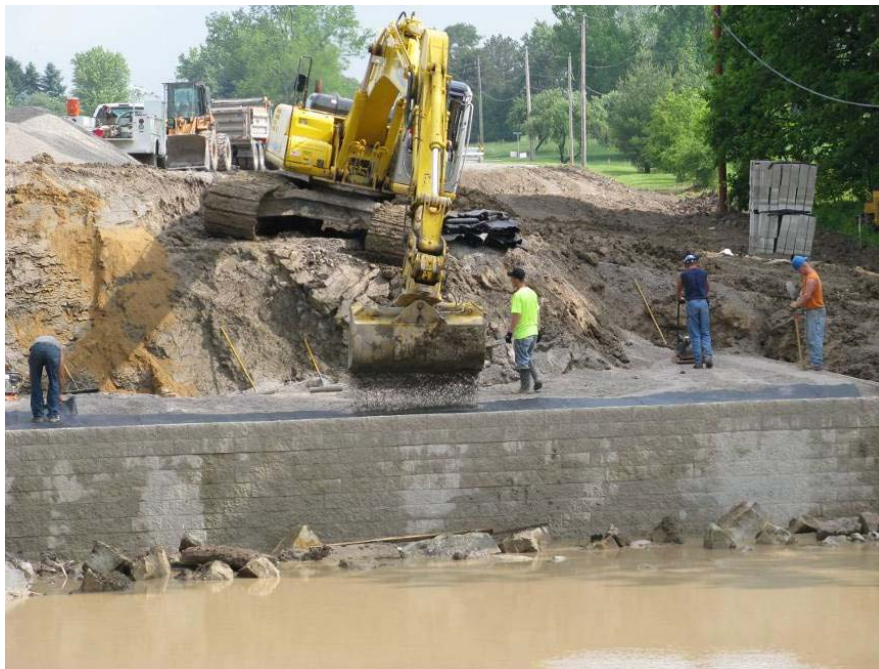
Figure 40. Photo. Typical labor crew with centrally located track hoe.
