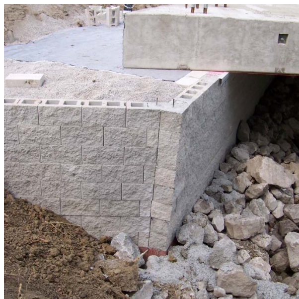
Figure 58. Photo. Vertical seam in wing wall.
