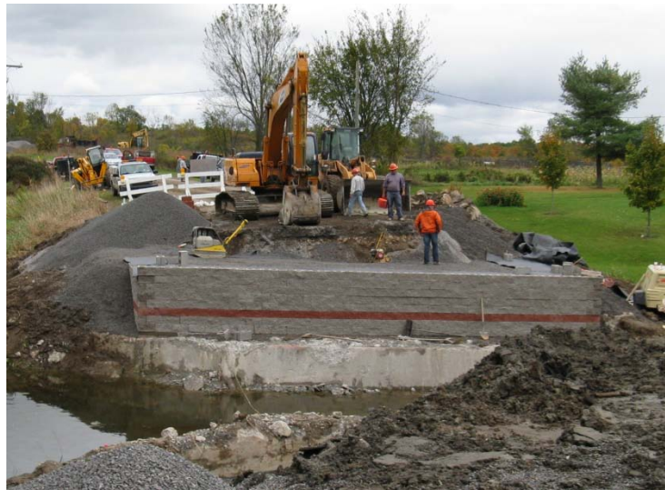
Figure 41. Photo. Cut slope of retained soil.
