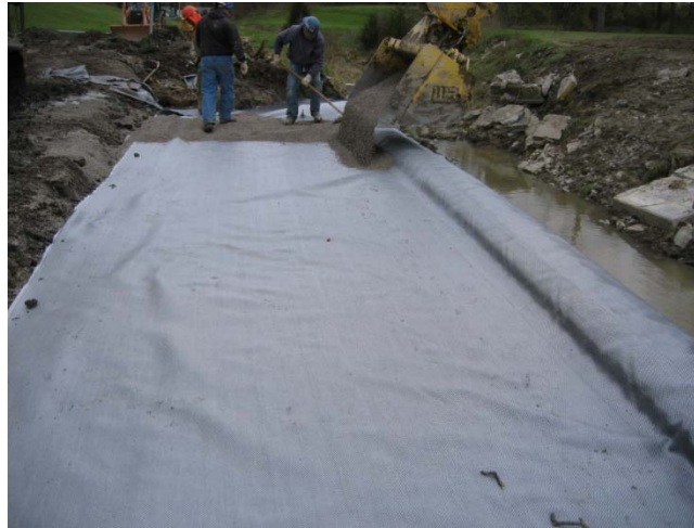
Figure 68. Photo. First 4-inch wrap butted against foam board.
