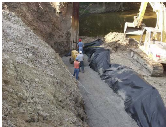
Figure 48. Photo. Encapsulation of fill in RSF.
