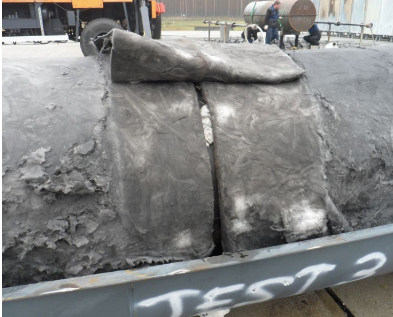
Figure 20. Test 3 - Second Layer of Insulation. Note the condition of the protected insulation
