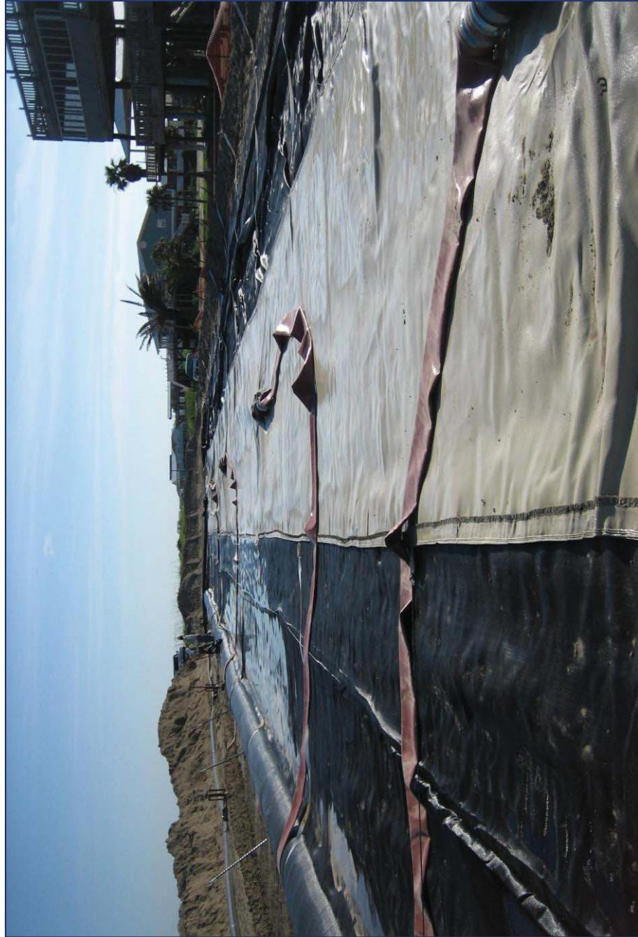
In severe erosion conditions, the width of the apron may be extended or circumference of anchor tube increased.
