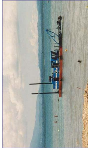
Dredging is the most common method of filling tubes.
