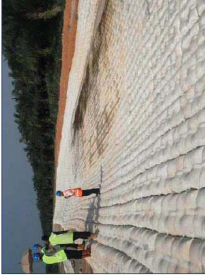
Geotextile mattresses placed over prepared slope.
