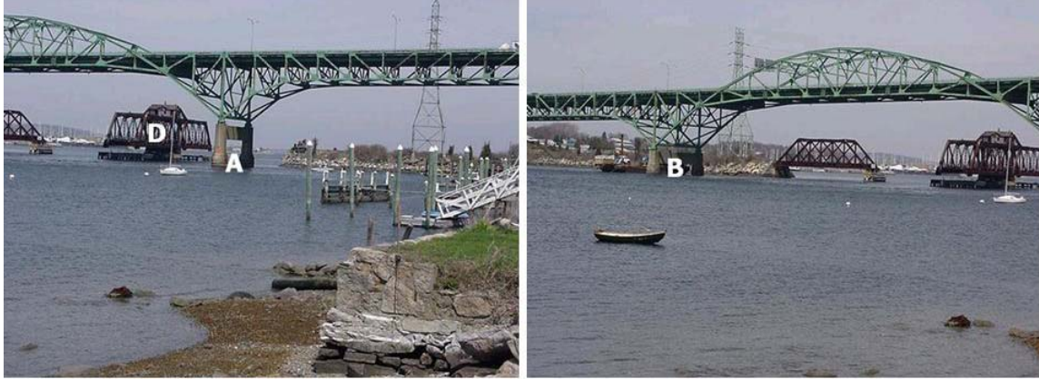
FIGURE 19. View of the highway bridge at Sakonnet with piers marked as A, B and D. The drilling barge (near B) and the old railroad bridge can also be seen in the picture.
