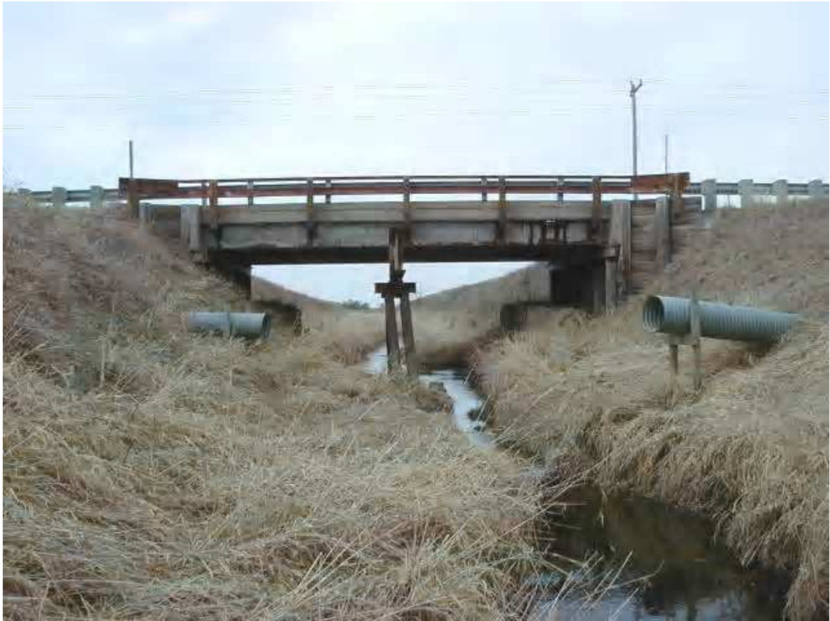
Figure 8.2. HCB Elevation View of Bridge Looking North.
