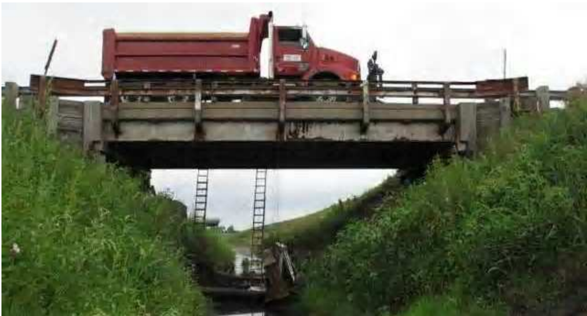
Figure 8.4. HCB Test Truck Crossing Bridge After Pier Removal.
