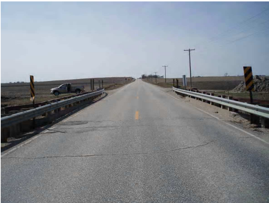
Figure 8.1. HCB Alignment View Looking West.
