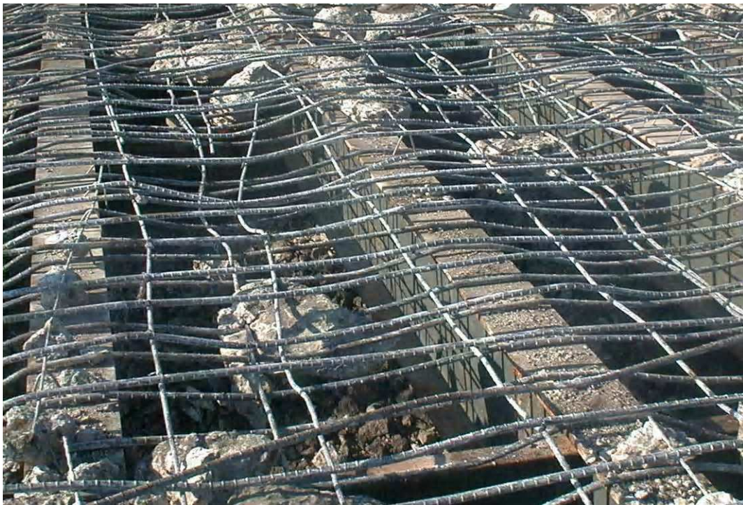
Figure 4.17. Exposed Top Flanges After MCB Deck Demolition.
