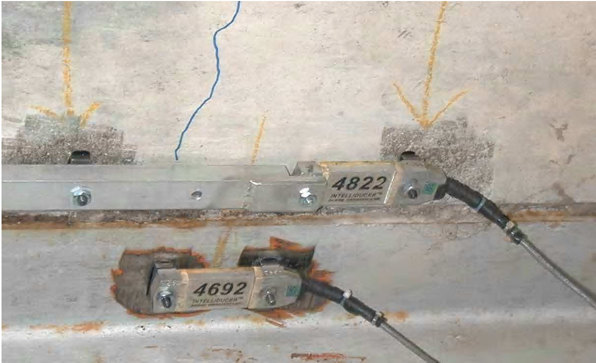
Figure 3.15. Concrete and Steel Mounted Transducers at Midspan of BCB.
