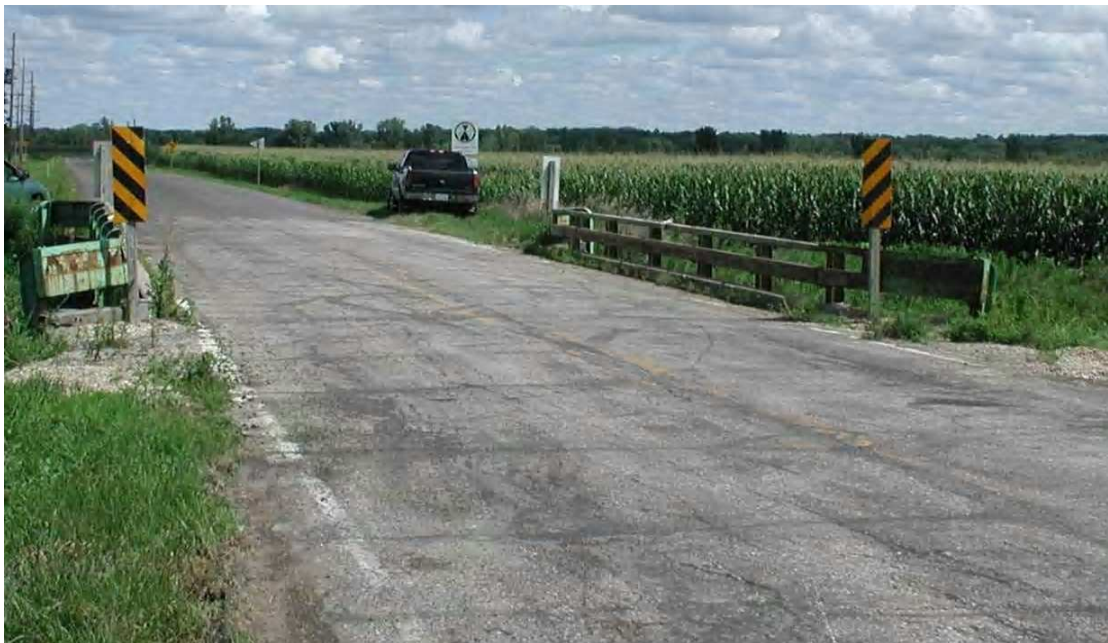
Figure 4.1. MCB Alignment View Looking North.
