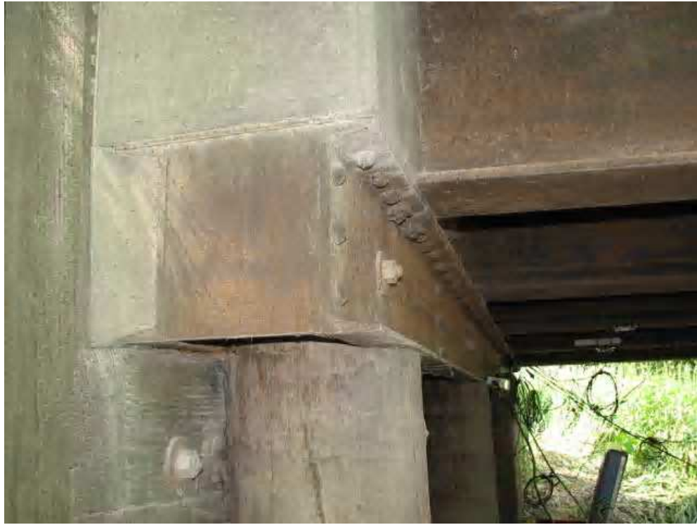
Figure 3.2. Typical Pile Cap Configuration.
