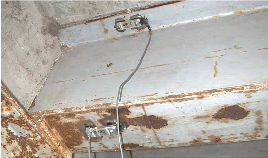
Figure 3.12. Instrumentation Near Abutment of BCB
