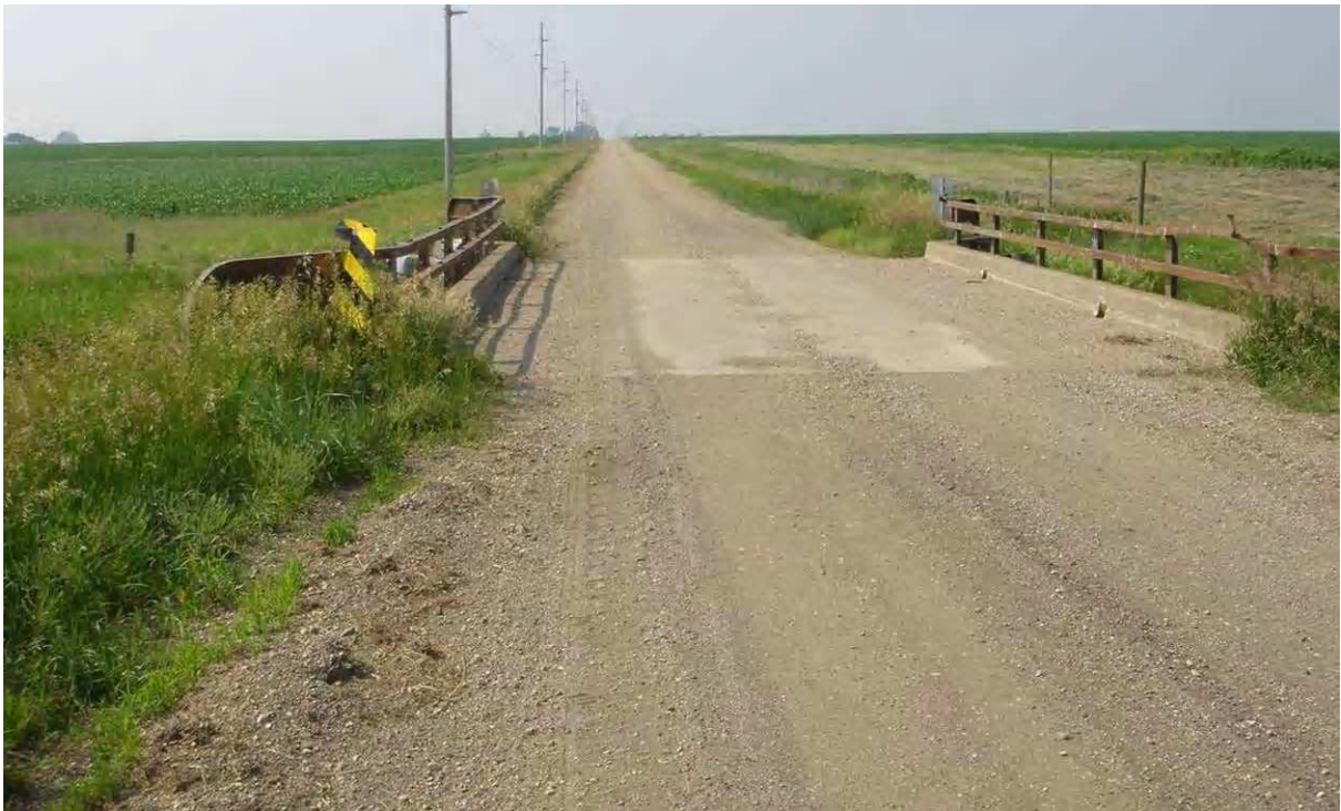
Figure 3.1. BCB Alignment View Looking South.
