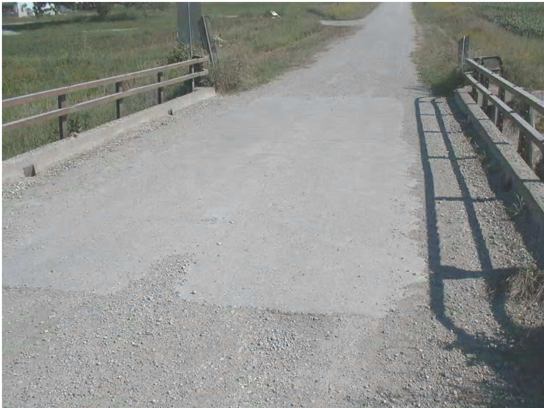
Figure 5.1. KCB1 Alignment View Looking North.
