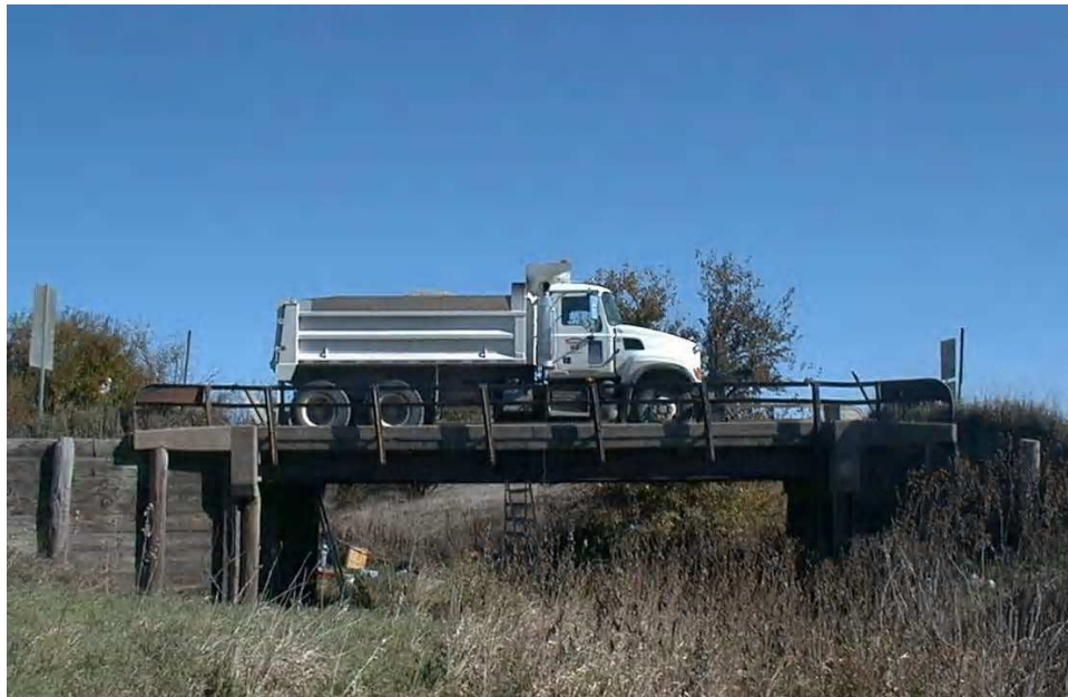
Figure 5.5. KCB1 Test Truck.
