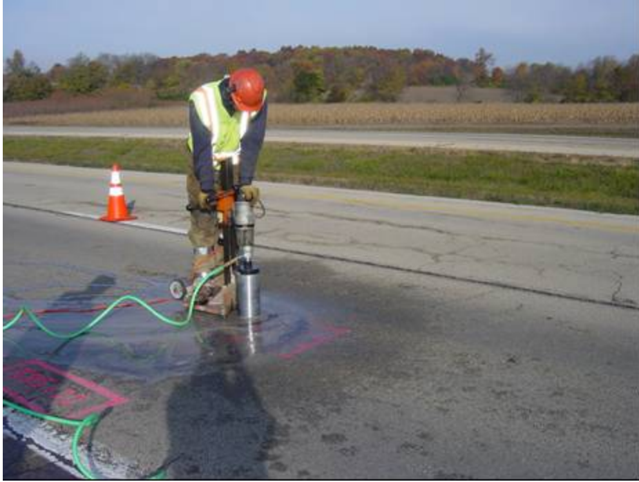
Figure D-2. Coring operation
