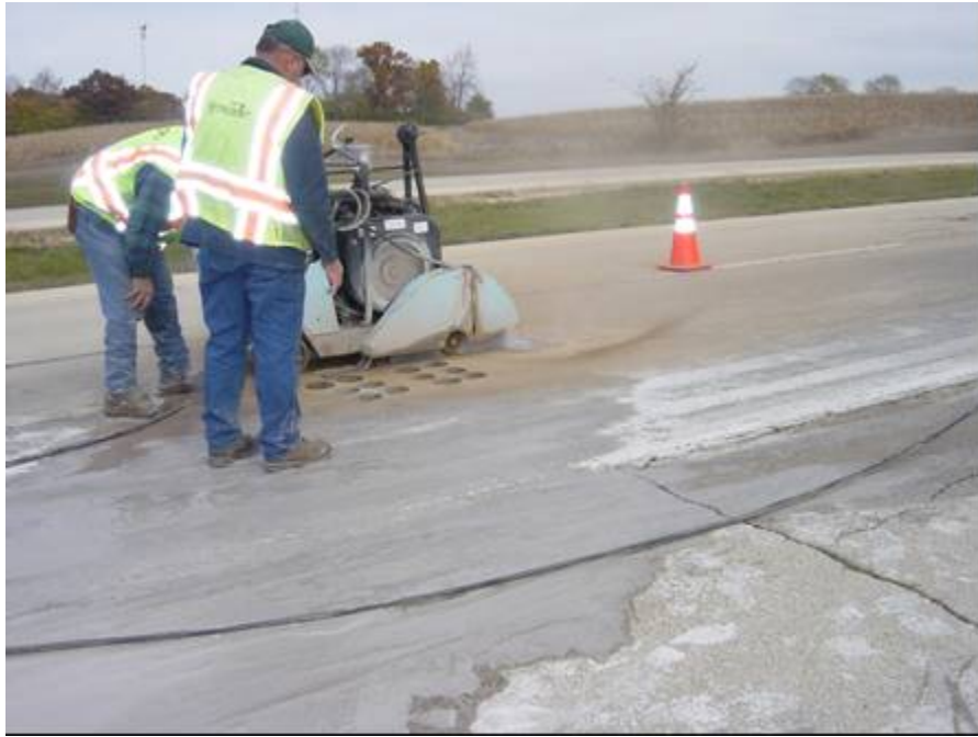
Figure D-4. Saw cutting
