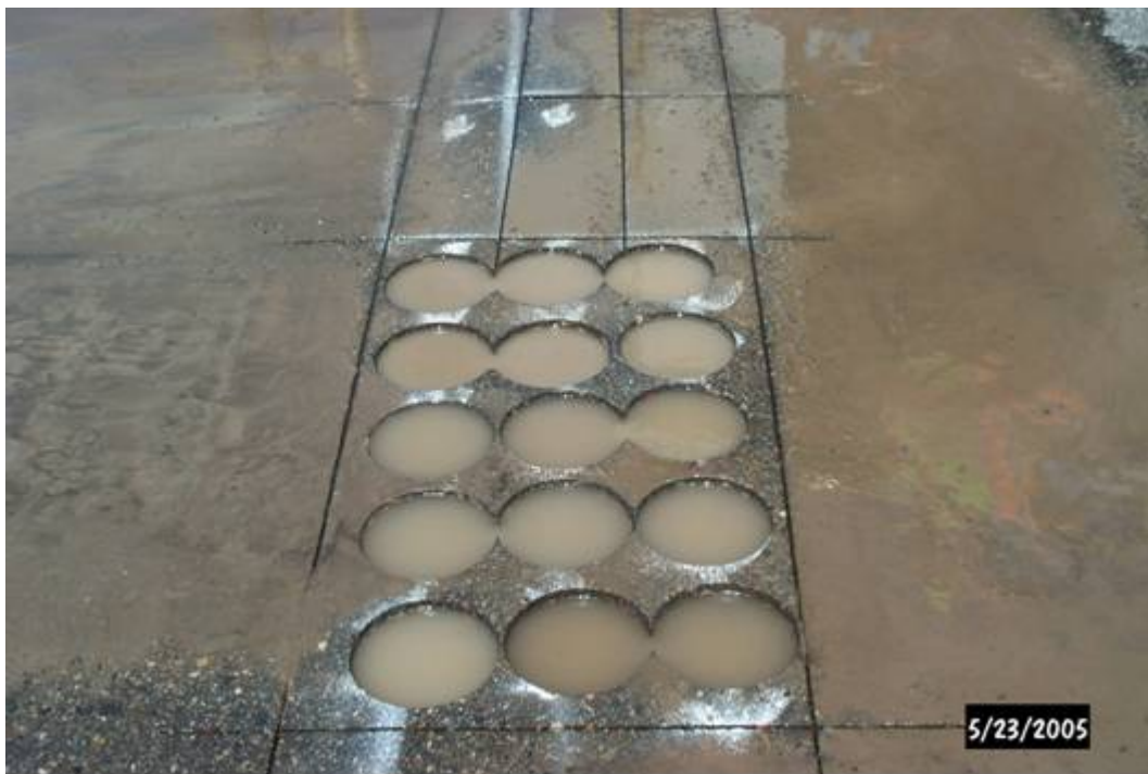
Figure C-4. Sample area after coring and cutting
