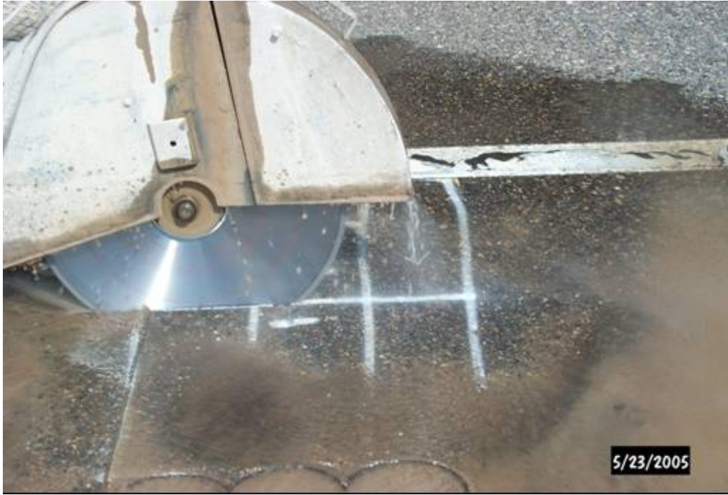
Figure C-3. Saw cutting beam samples
