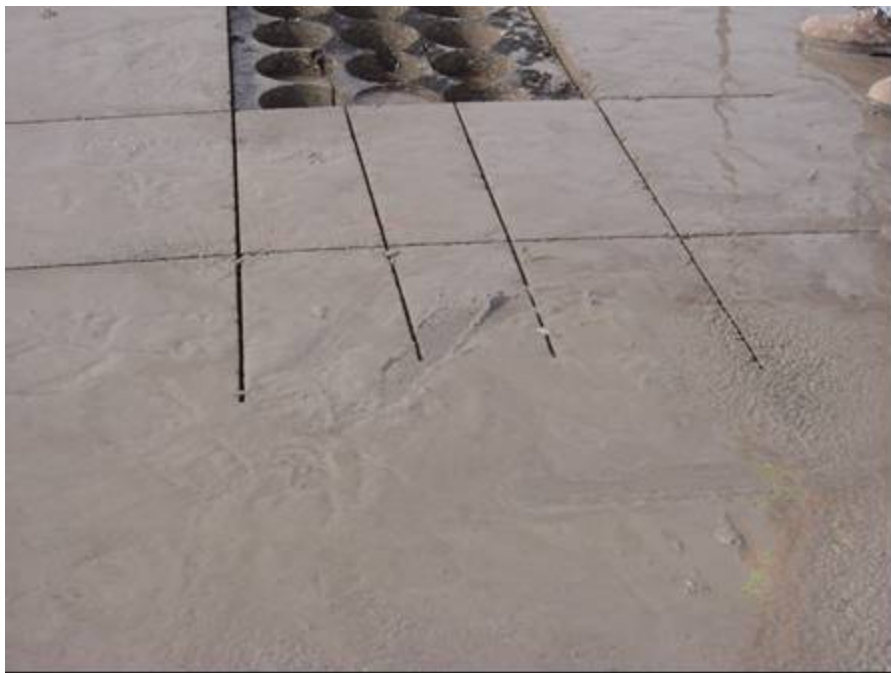
Figure D-5. Cut beams in road
