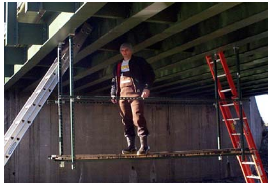
FIGURE 1: Scaffolding Used in January Test
