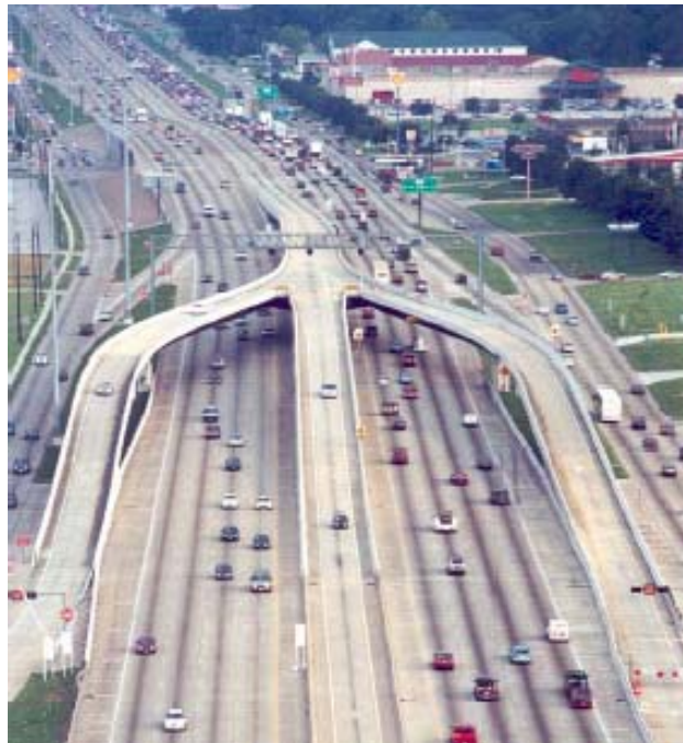
Figure 9. Direct Access Ramp.
