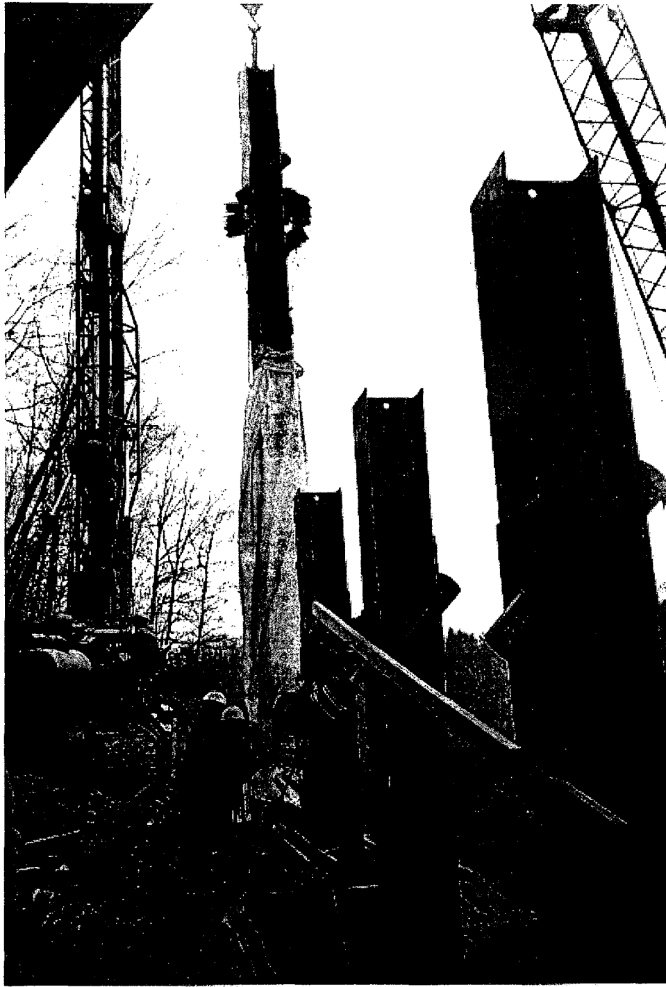
Fig 3.34: The soldier pile being wrapped with plastic sheet to prevent contact with concrete.
