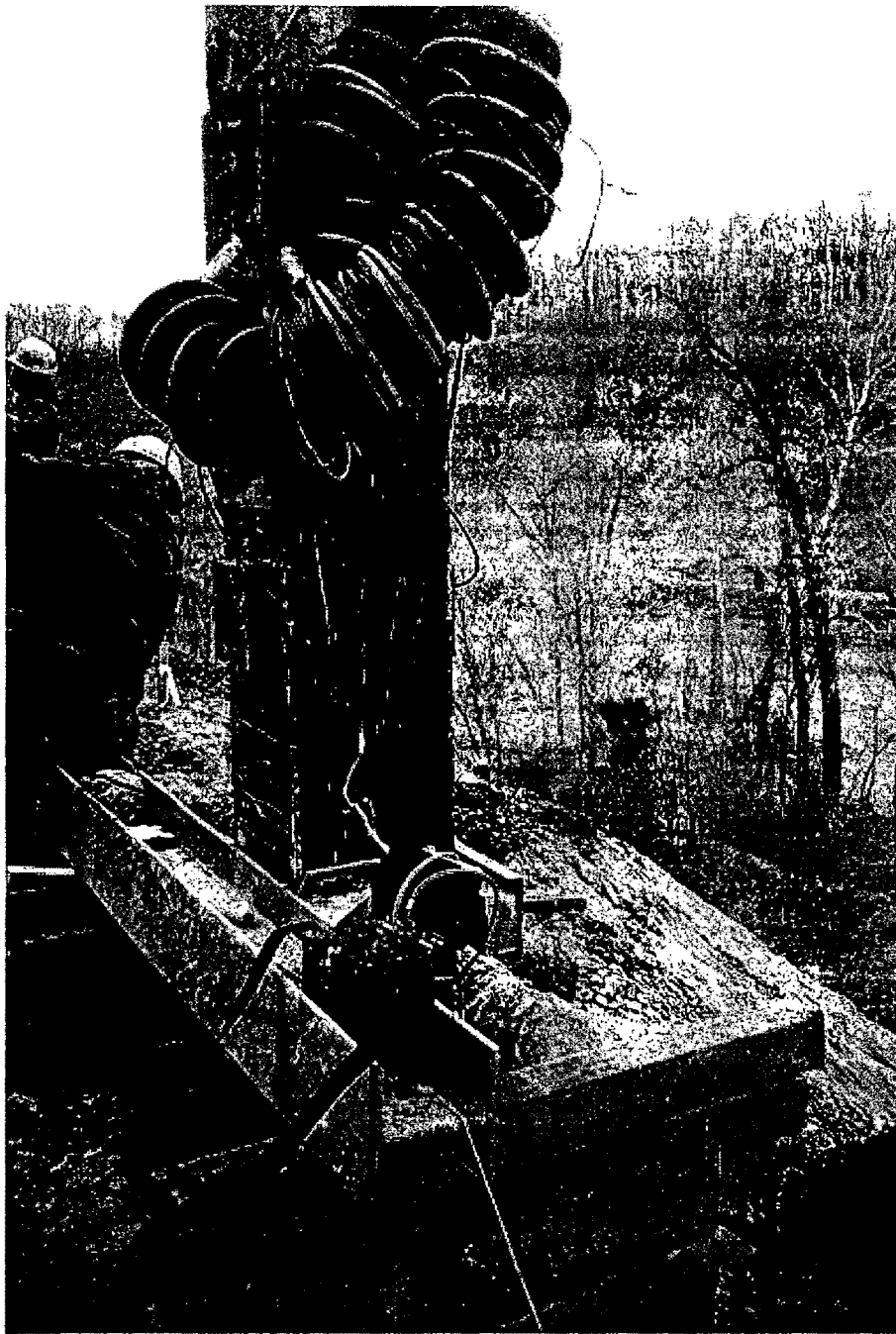
Fig 3.36: The strain gages being checked after the pile was installed.
