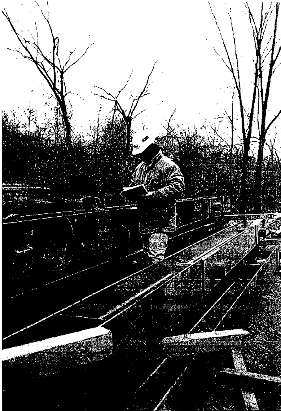
Fig 3.11: A series of gages being installed and checked.
