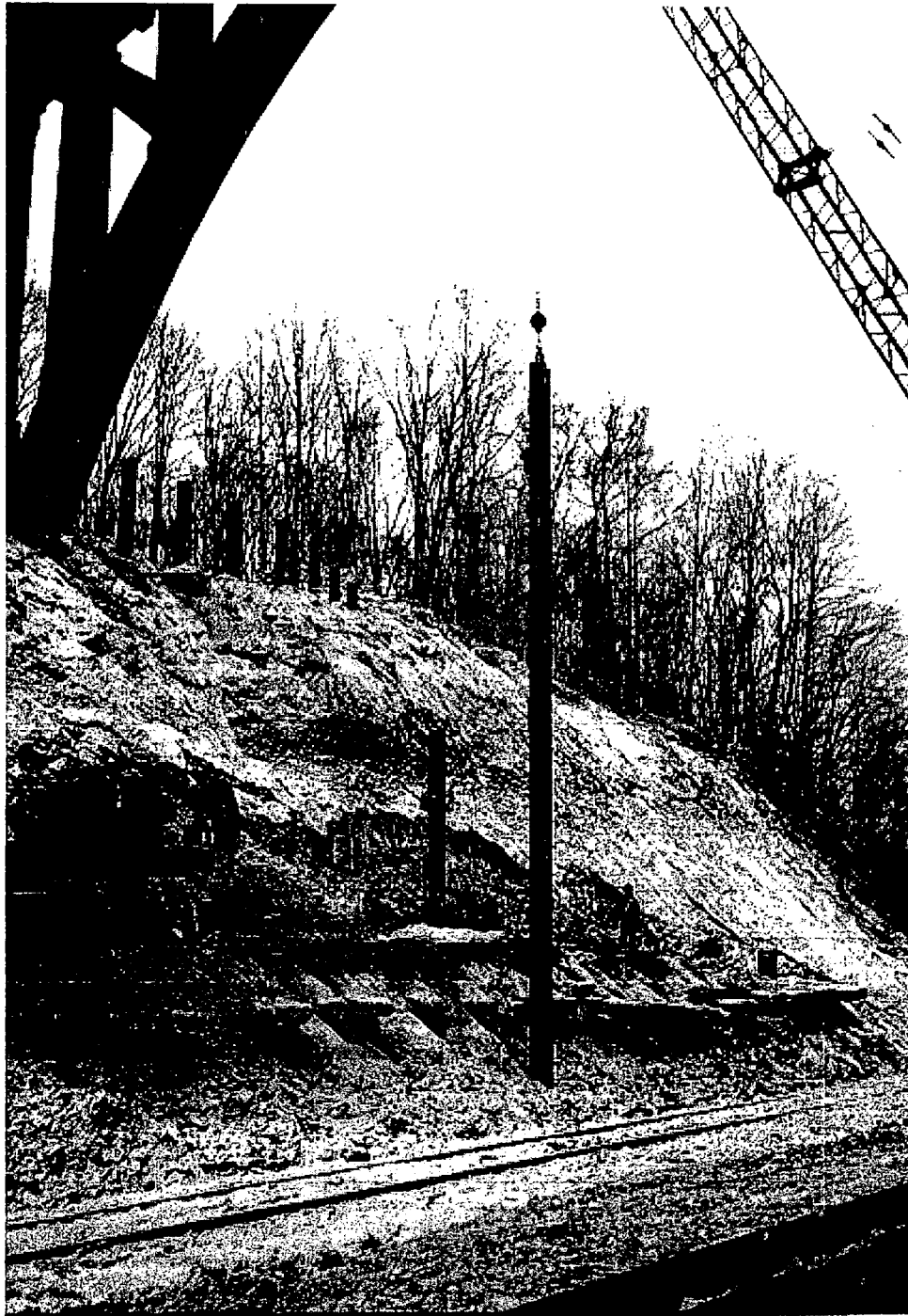
Fig 3.31: Instrumented soldier pile being lifted for installation.
