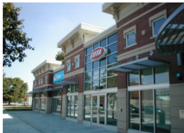
Figure 21: Near East Transit Center
