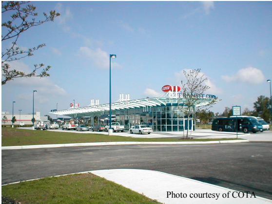
Figure 23: Easton Transit Center
