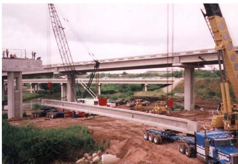
Figure 7.3-1 Long-span Prestressed Concrete Beam Erection
