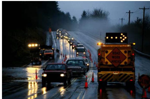
Figure 9. Work-Zone Conditions Affect Military Deployments, Which May Inhibit General Traffic Operations
