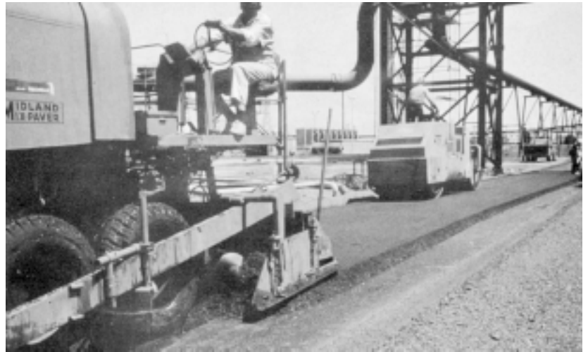
A mix paver placing cold recycled mix.
