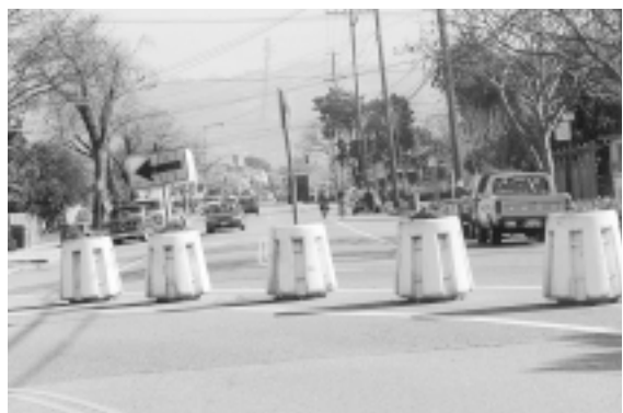
Route modifications such as diagonal diverters, top and bottom, and partial diverters, middle, should only be installed after extensive study of possible spillover effects.
