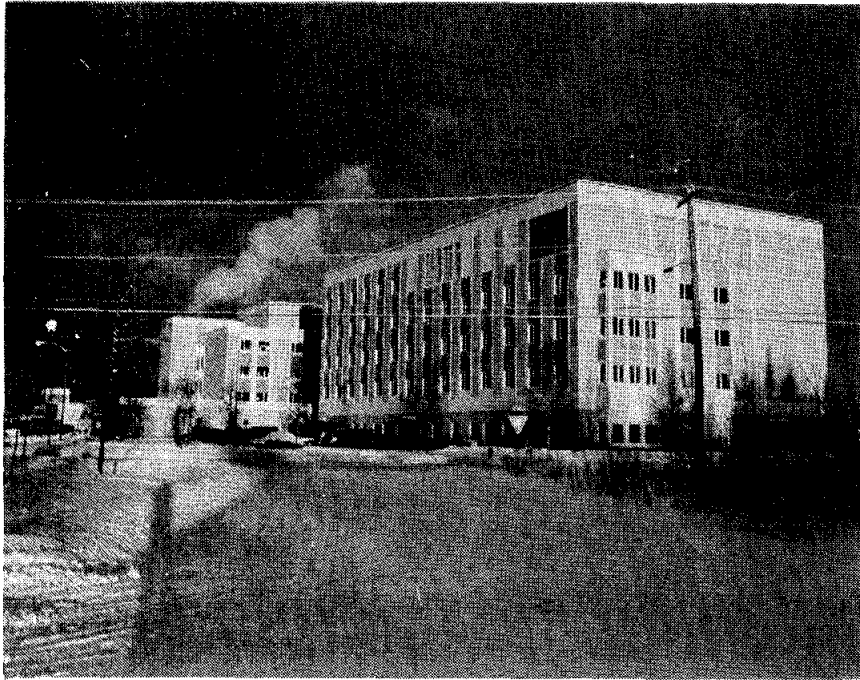
Figure 5 - Fairbanks Memorial Hospital, 1650 Cowles Street
