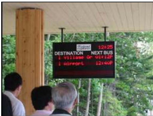
Figure 4.4: Electronic Bus Departure Sign at Visitor Center
