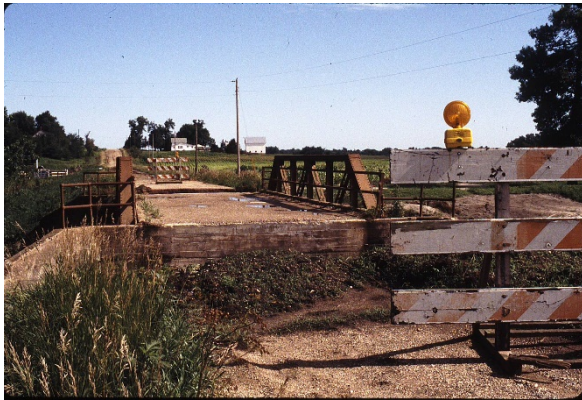
Figure 1.1 Effect of flood on erosion at a small bridge with two (wing-wall) abutments situated in Squaw Creek, close to Ames (Iowa).
