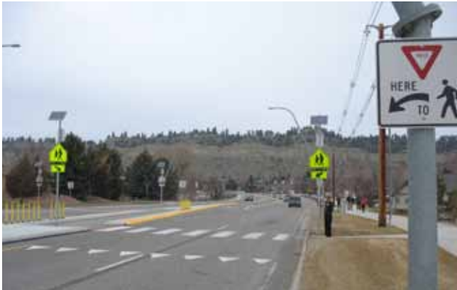
RRFB crossing of Shiloh Avenue in Billings
