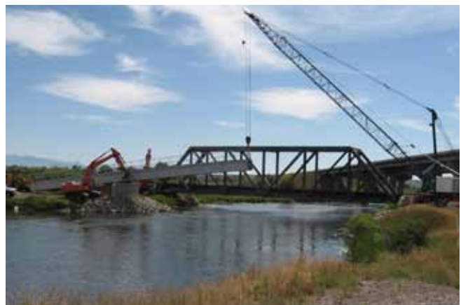
The 'recycled' bridge being hoisted into position
