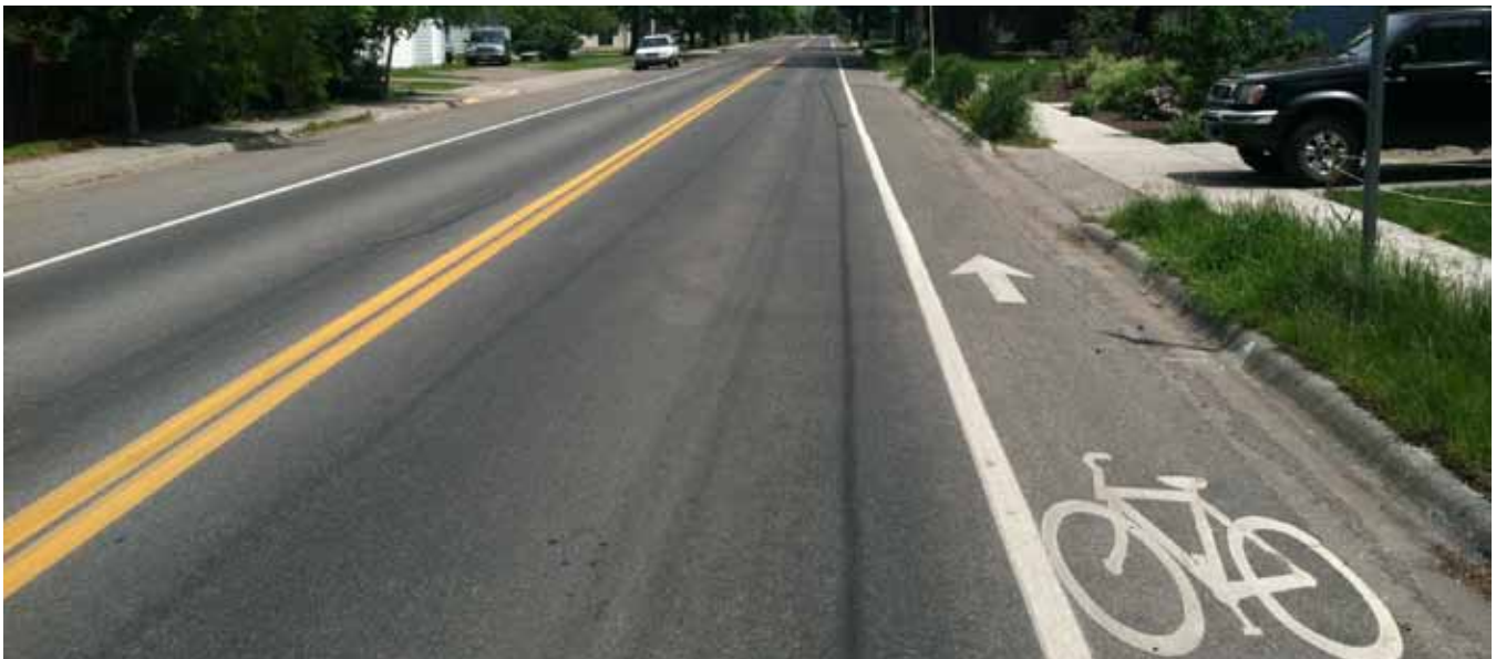
Parking removal for bike lane on Peach Street in Bozeman
