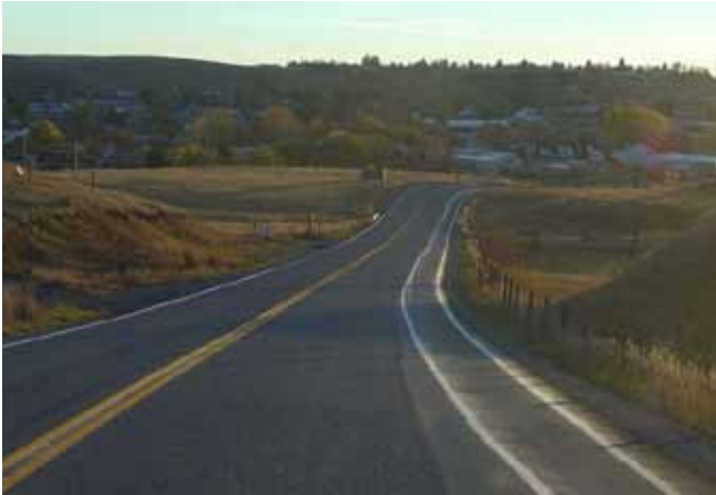
Shoulder bikeway near Shelby - Note: shoulder not chip sealed
