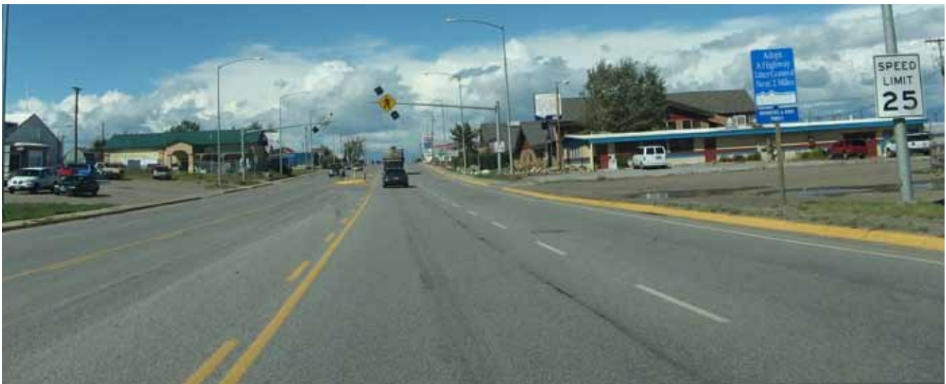
This arterial has sufficient curb-to-curb and overall right-of-way to accommodate bike lanes and sidewalks
