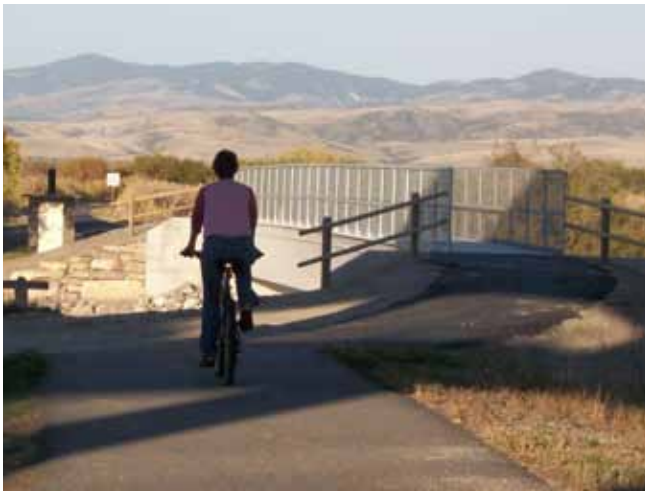
Completed bridge over the Madison River
