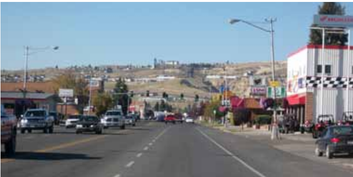
Harrison Avenue in Butte, MT before reconstruction
