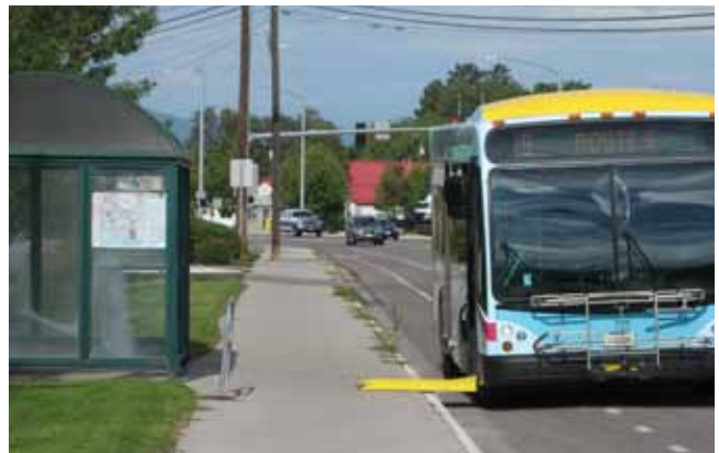
In Missoula, this sidewalk acts as a maneuvering space for disabled users
