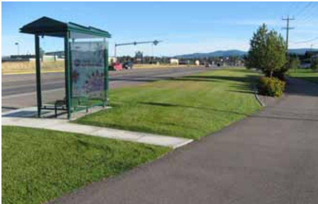
Transit stop with good pedestrian/disabled access
