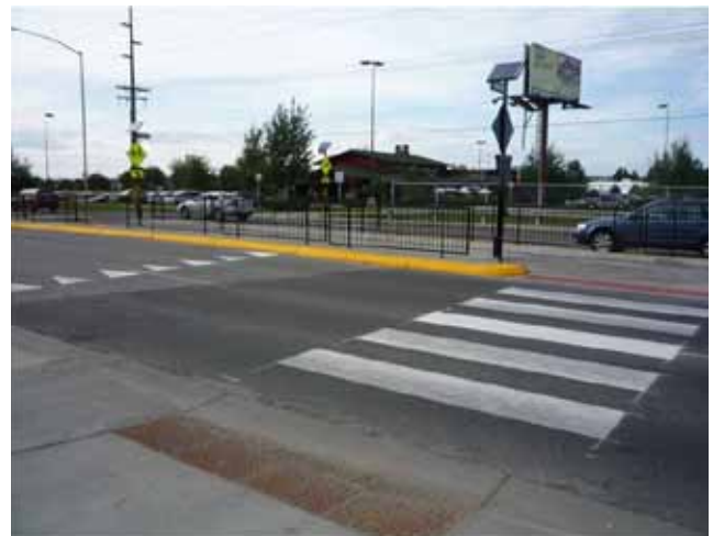
RRFB on King Avenue West in Billings
