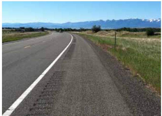
Well designed rumble strip
