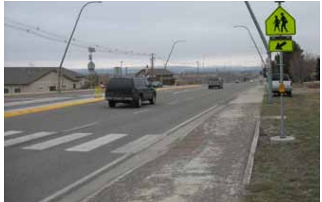
RRFB crossing in Billings - Note debris on sidewalk
