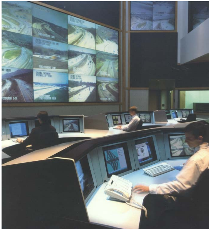
Figure 3.13 CCTV Display Wall in TOC
