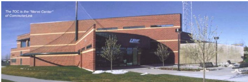
Figure 3.1 Traffic Operations Center
