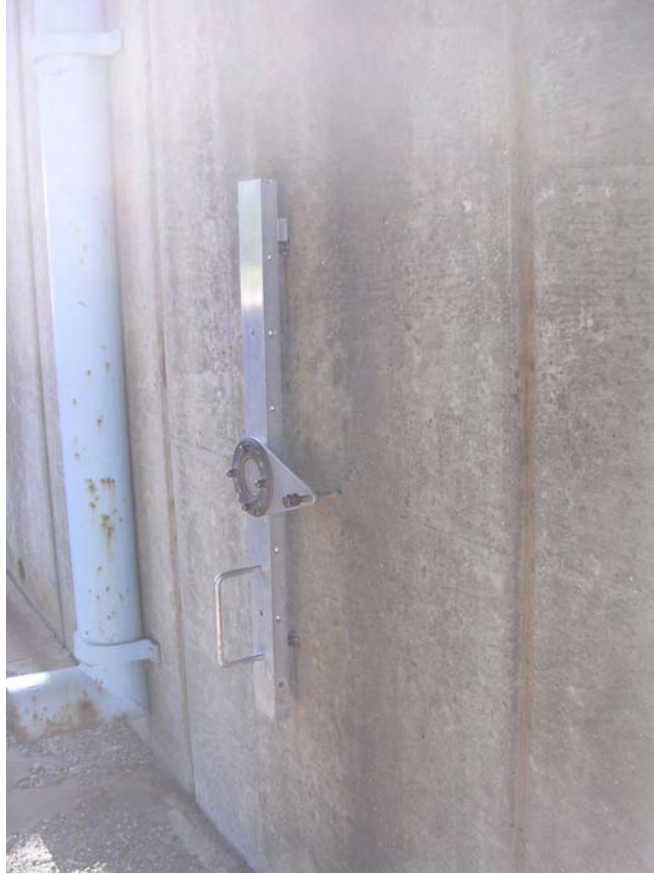
Figure 2.4: Reference Plate Attached to Wall Panel
