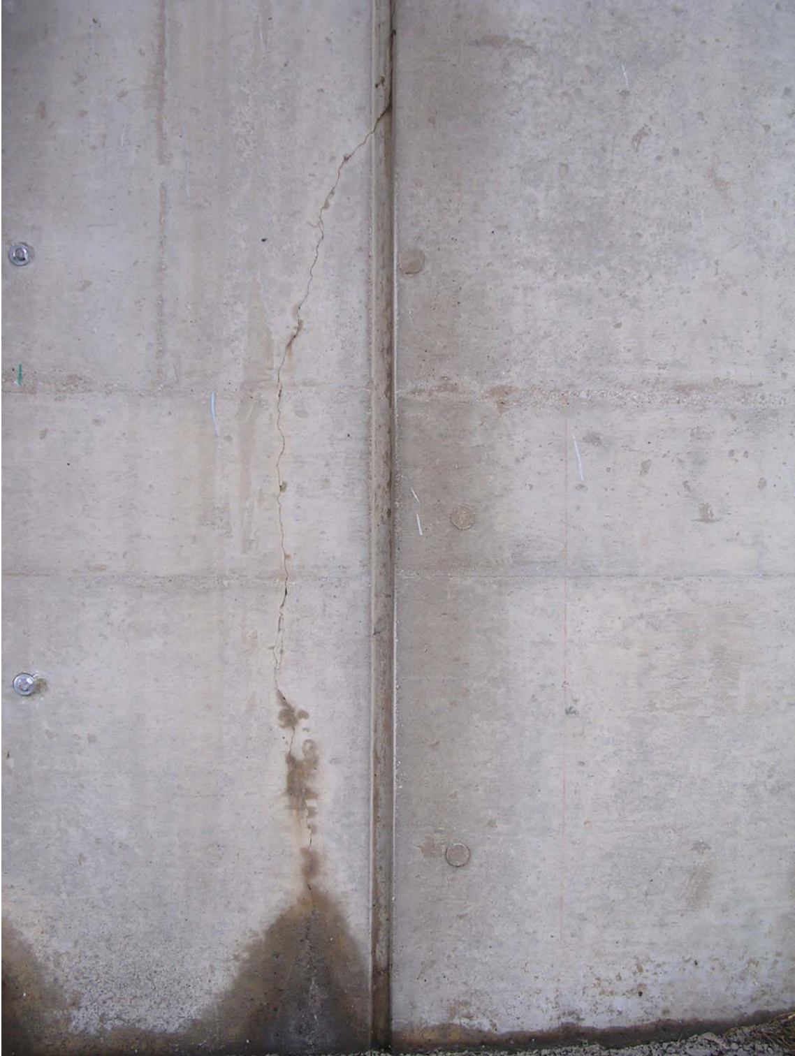
Figure 3.13: General View of Panel N-2
