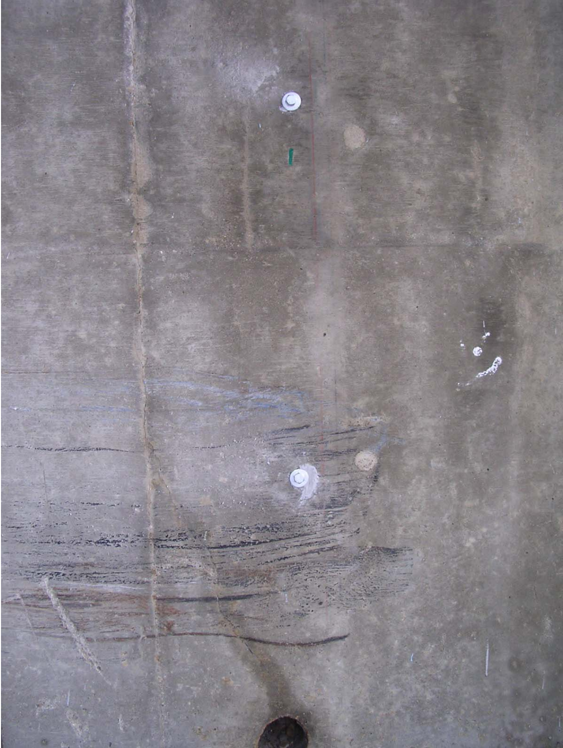
Figure 3.7: General View of Panel S-1
