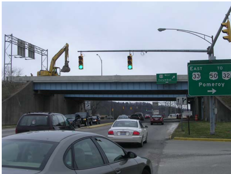
Figure 1.1: Project Site Area (SR 33 over E. State St. – Athens)
