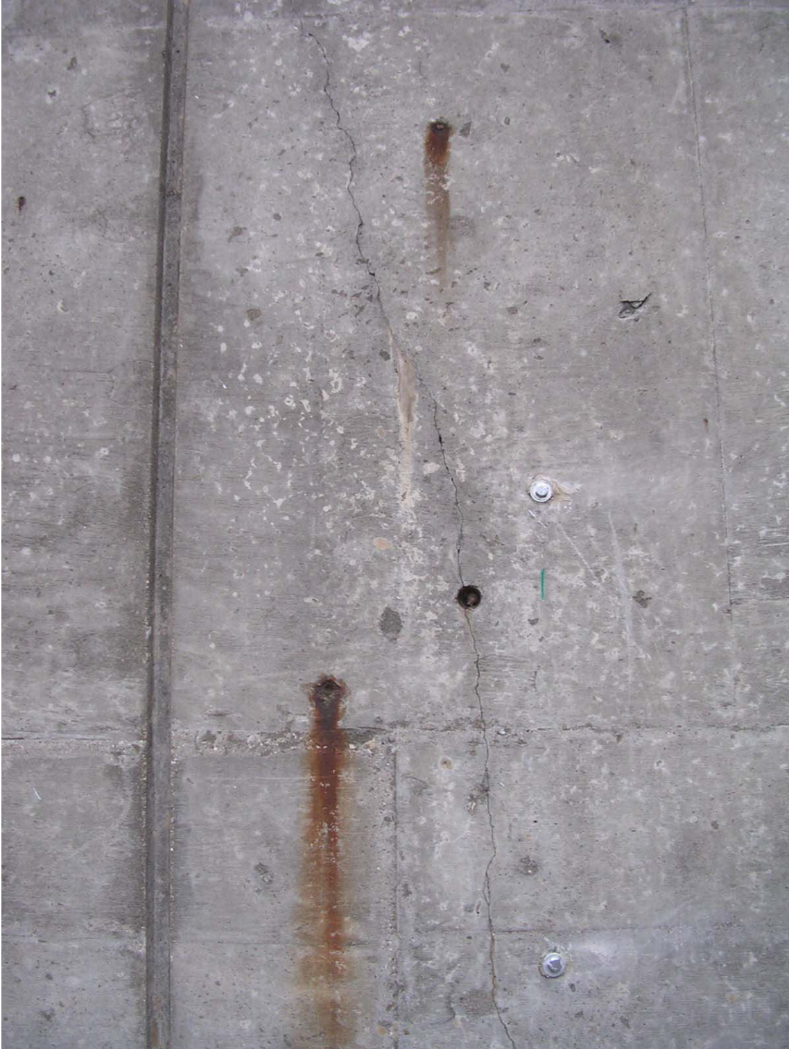
Figure 3.15: General View of Panel N-3
