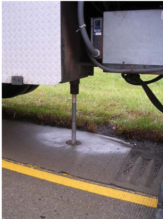
Figure 3.1: CPT Probe Pushed into Ground at Hole #1
