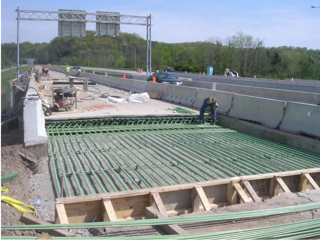
Figure 3.31: Reconstruction of Bridge Deck End Section
