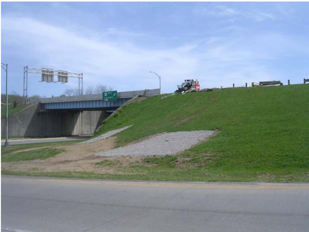
Figure 3.30: General View of Finished Drain Pipe Installation Work
