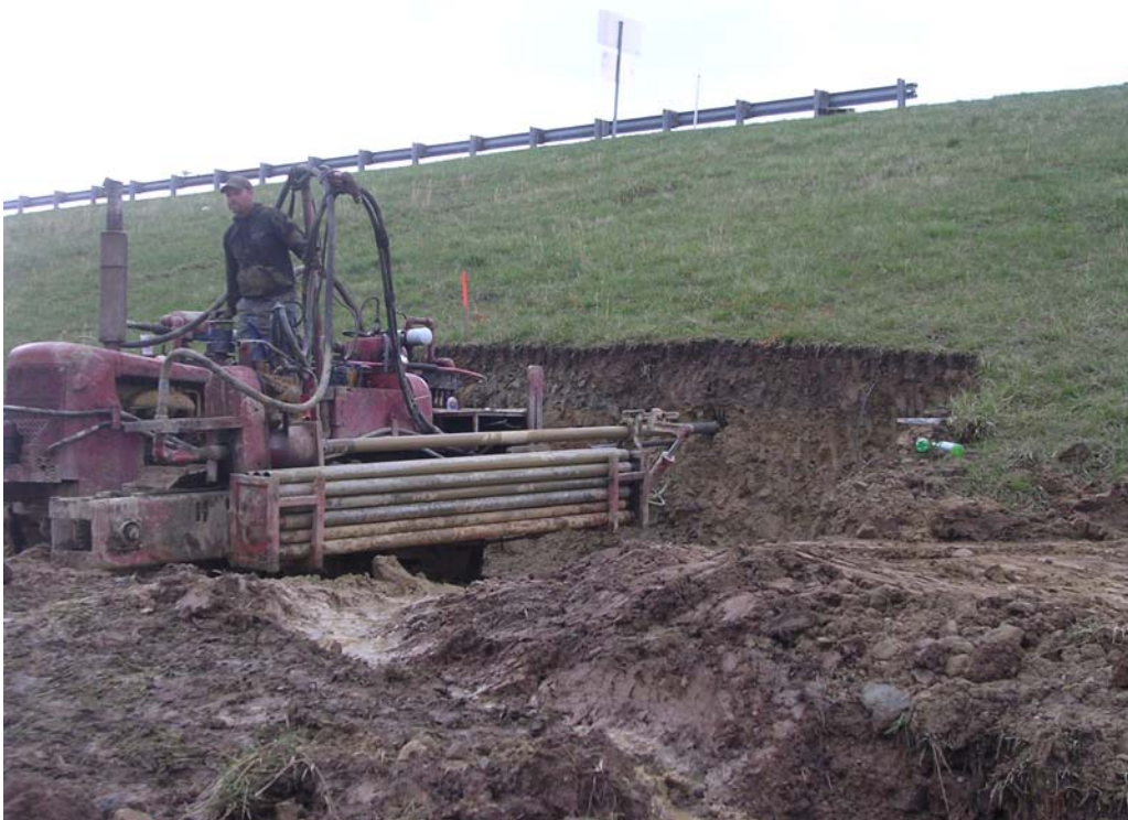
Figure 3.28: Horizontal Drain Pipe Installation Process
