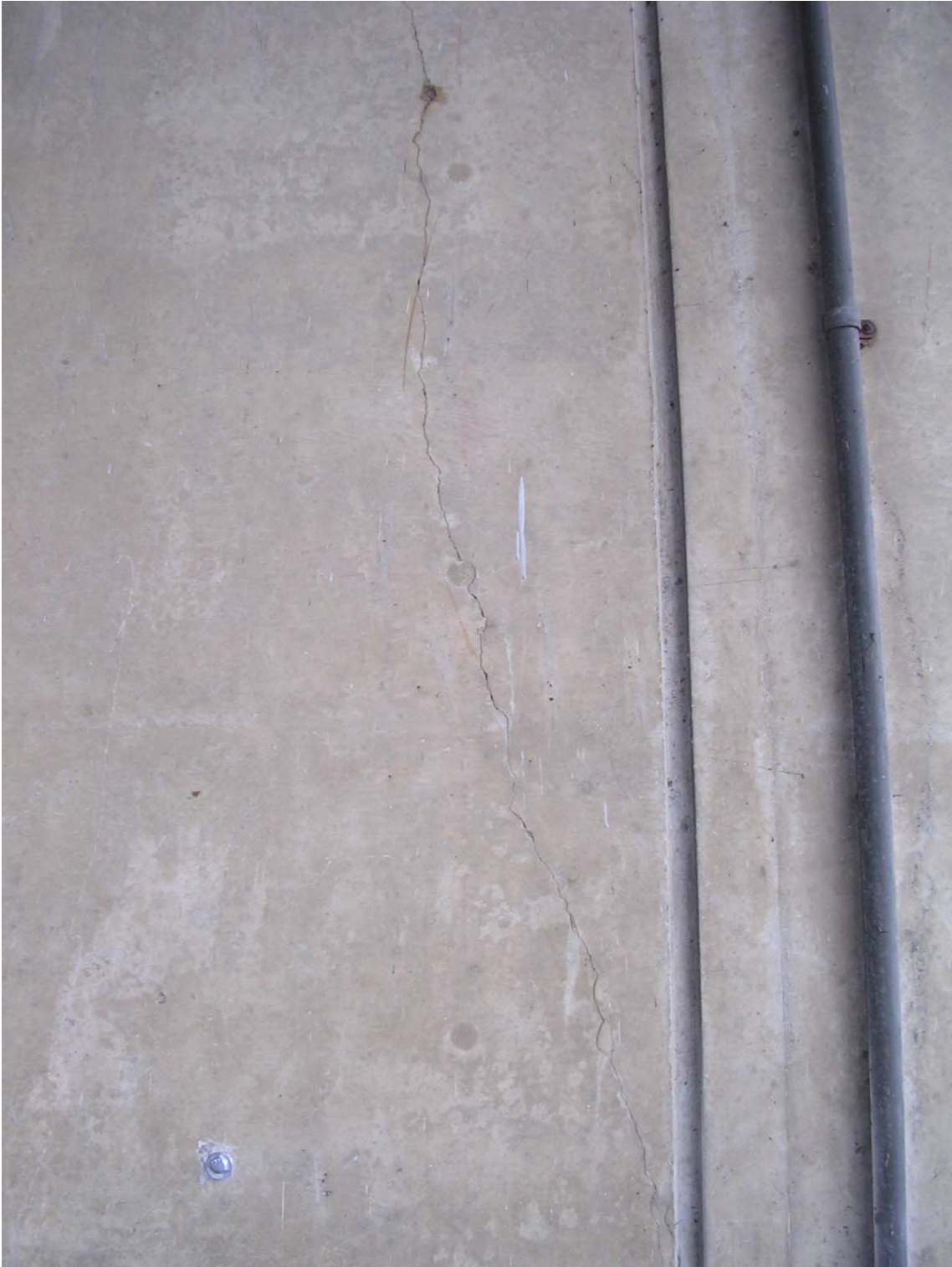
Figure 3.20: General View of Panel N-5 (Photo B)
