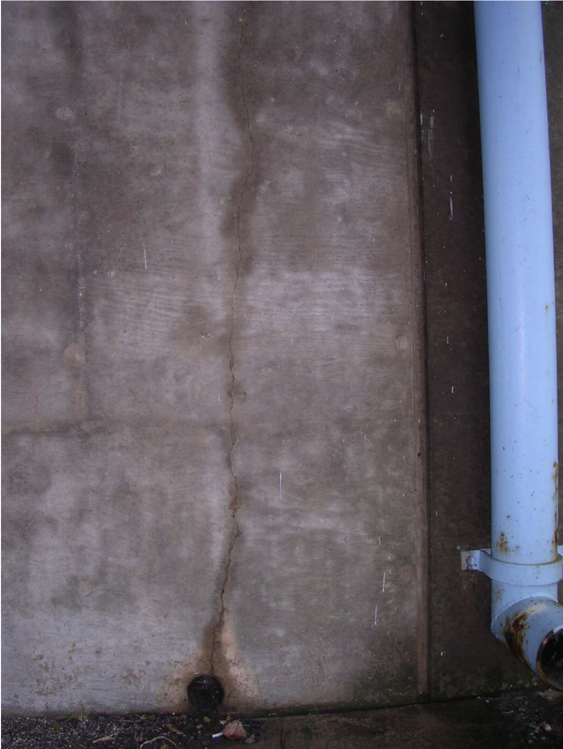
Figure 3.9: General View of Panel S-4
