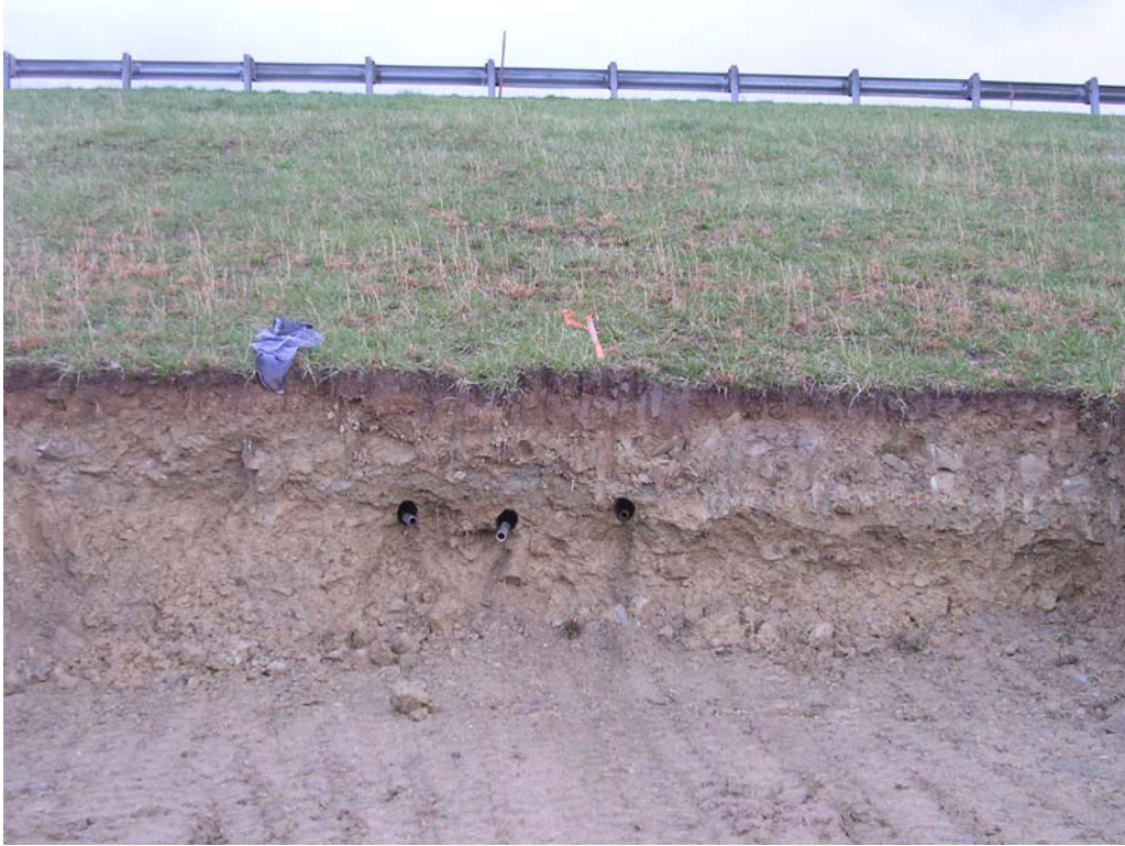
Figure 3.29: General View of Drain Pipes Installed at Sta. 819+75
