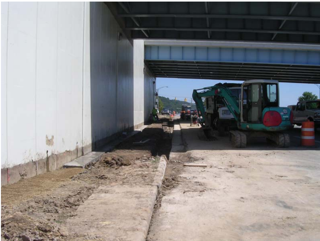
Figure 3.32: Construction of Sidewalk on North Side of E. State St.
