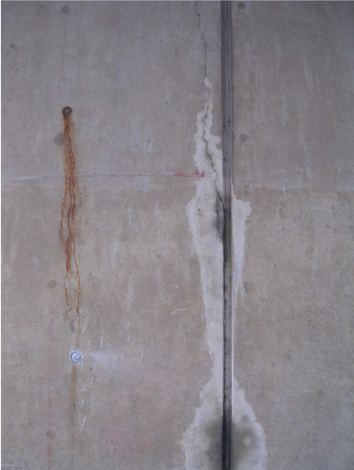
Figure 3.18: General View of Panel N-4 (Photo B)
