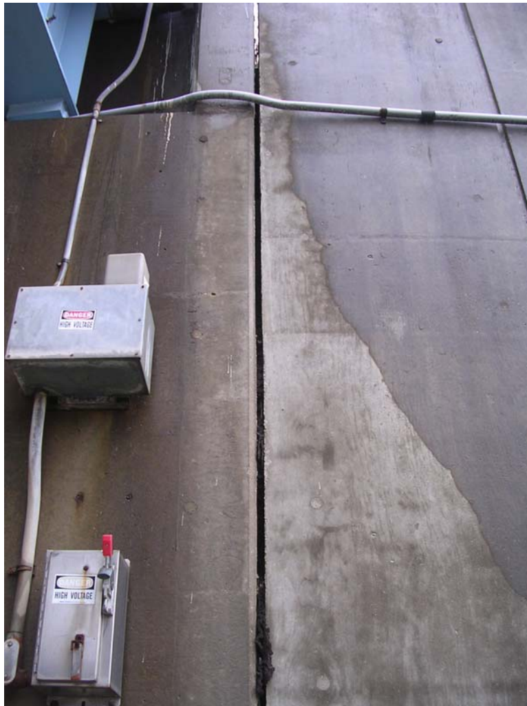
Figure 3.6: General View of Panel S-1 and SW Wingwall
