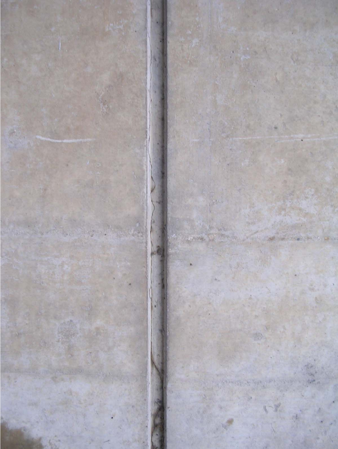
Figure 3.19: General View of Panel N-5 (Photo A)
