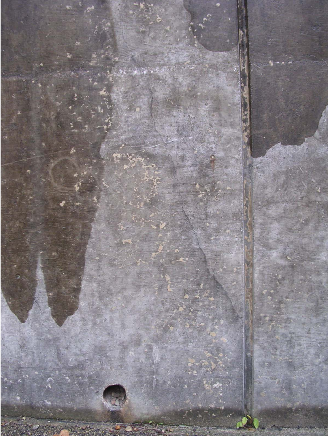
Figure 3.8: General View of Panel S-3
