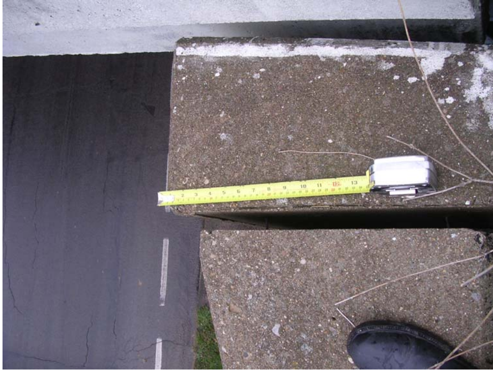
Figure 2.6: Taking Joint Measurements at Top of Abutment Wall
