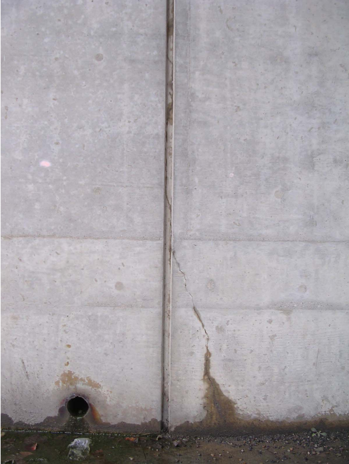
Figure 3.17: General View of Panel N-4 (Photo A)
