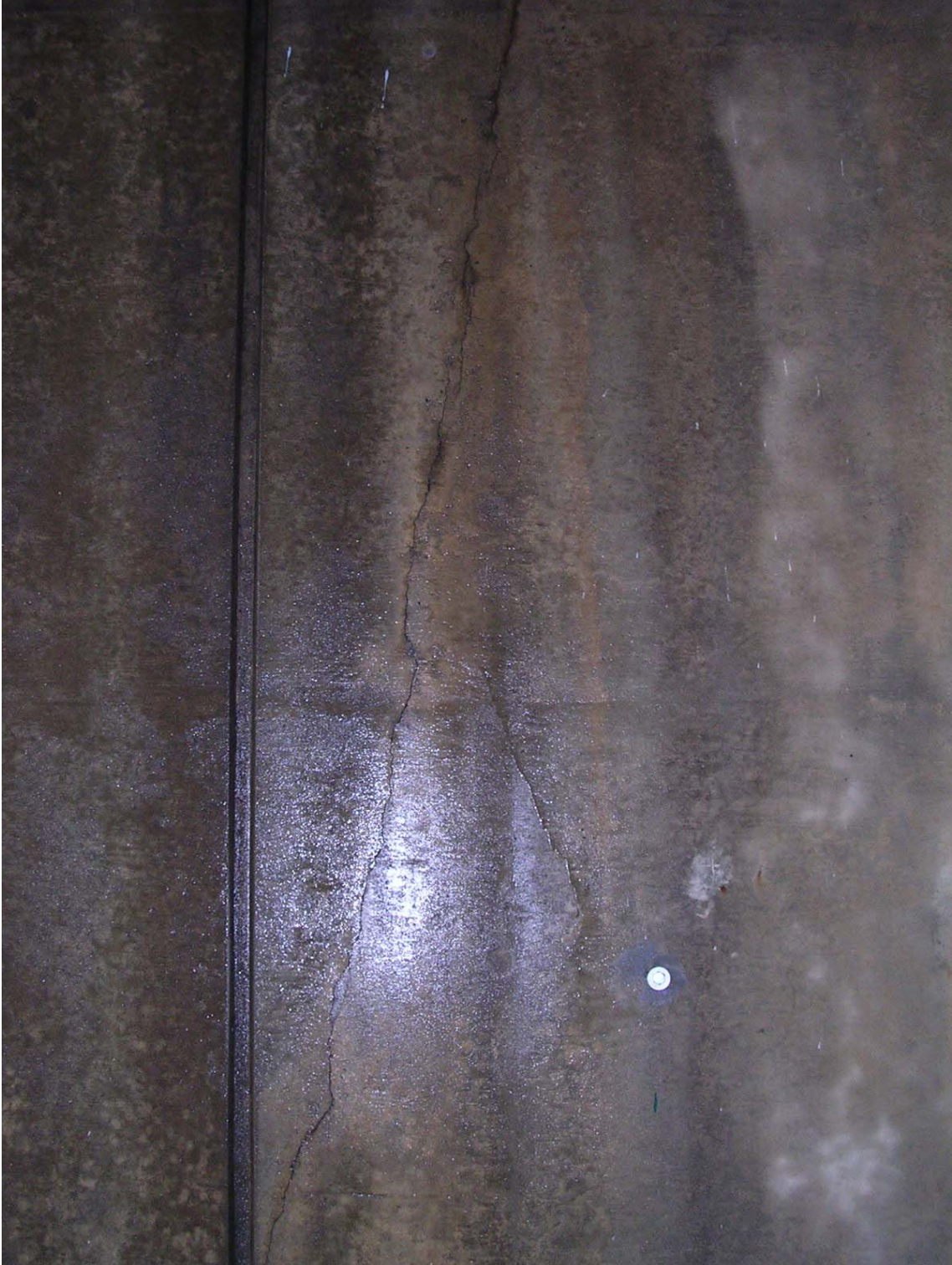
Figure 3.10: General View of Panel S-5
