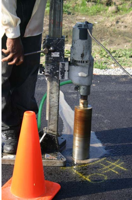
Figure 7.7 – Asphalt Coring
