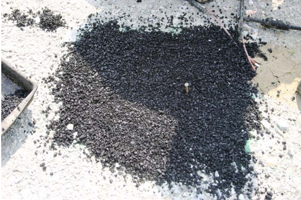
Figure 4.9 – Bottom Asphalt Cushion and Alignment Nail
