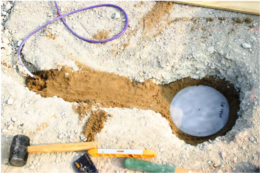
Figure 4.5 – Installed Base Course Earth Pressure Cell
