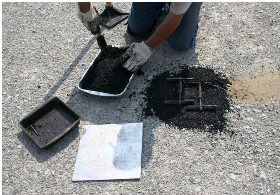
Figure 4.10 – Strain Gage Installation In Progress
