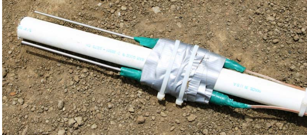
Figure 4.15 – Subgrade Thermocouples Attached to a PVC Pipe
