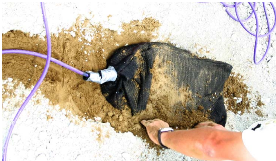
Figure 4.24 – Placement of the Piezometer
