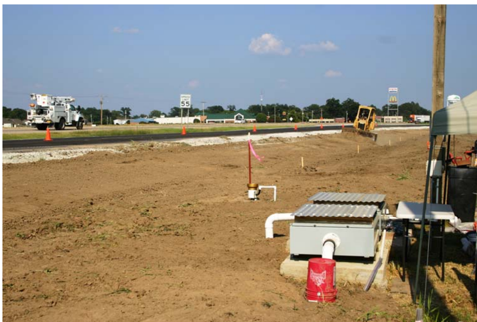
Figure 5.11 – Redressing the Side Slopes
