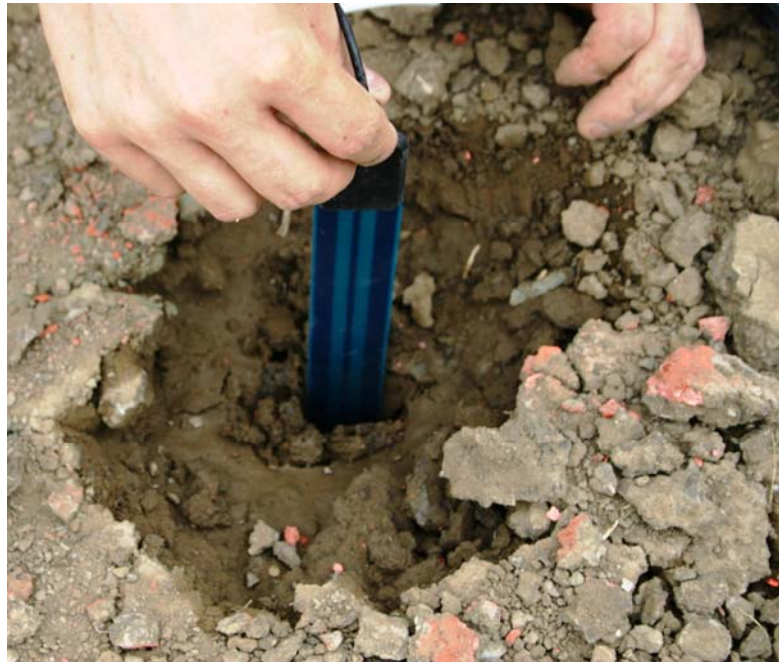
Figure 4.20 – Insertion of Subgrade Moisture Content Probe
