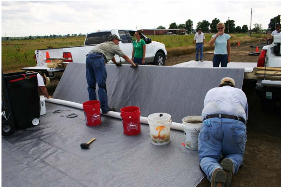
Figure 5.3 – Geosynthetic Lay Down Technique
