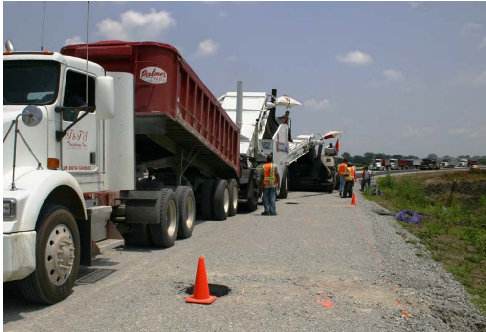
Figure 5.6 – Paving in Progress
