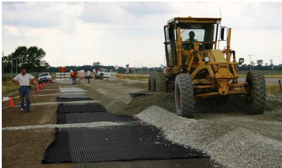
Figure 5.4 – Aggregate Placement
