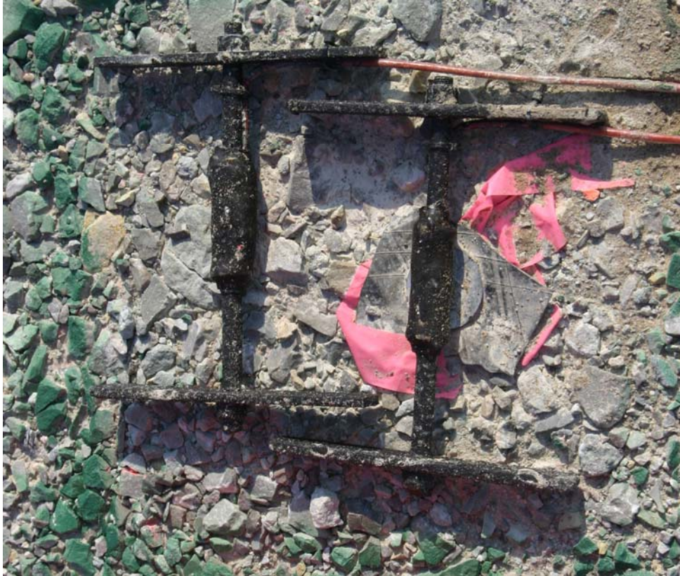
Figure 4.8 – Asphalt Strain Gage Pair Prior to Paving
