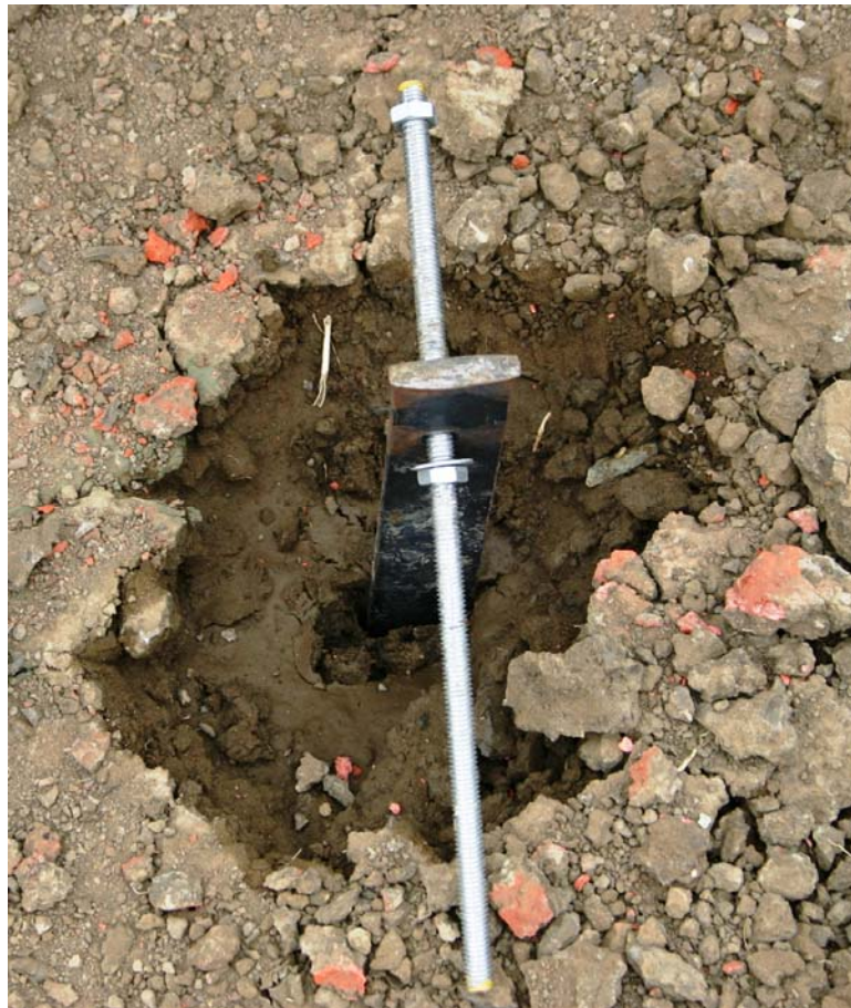
Figure 4.19 – Insertion of Metal Bar with Leverage Rod
