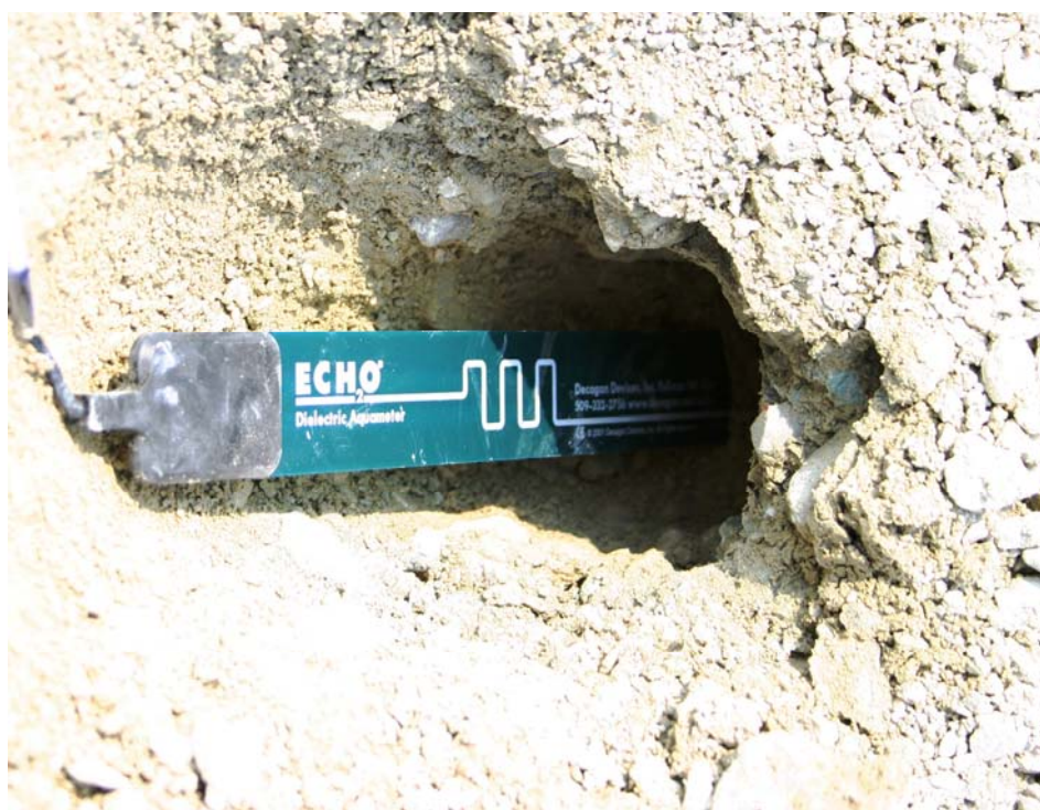
Figure 4.21 – Insertion of Base Course Moisture Content Probe
