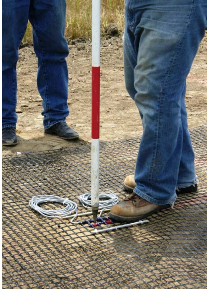
Figure 5.2 – Relocation of the Instrumentation Location
