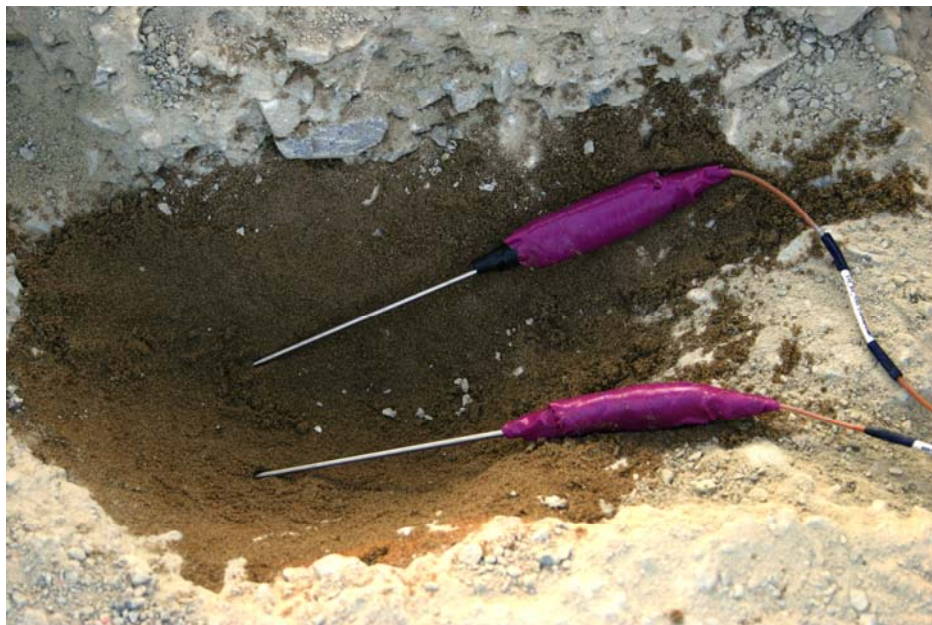
Figure 4.16 – Base Course Thermocouples
