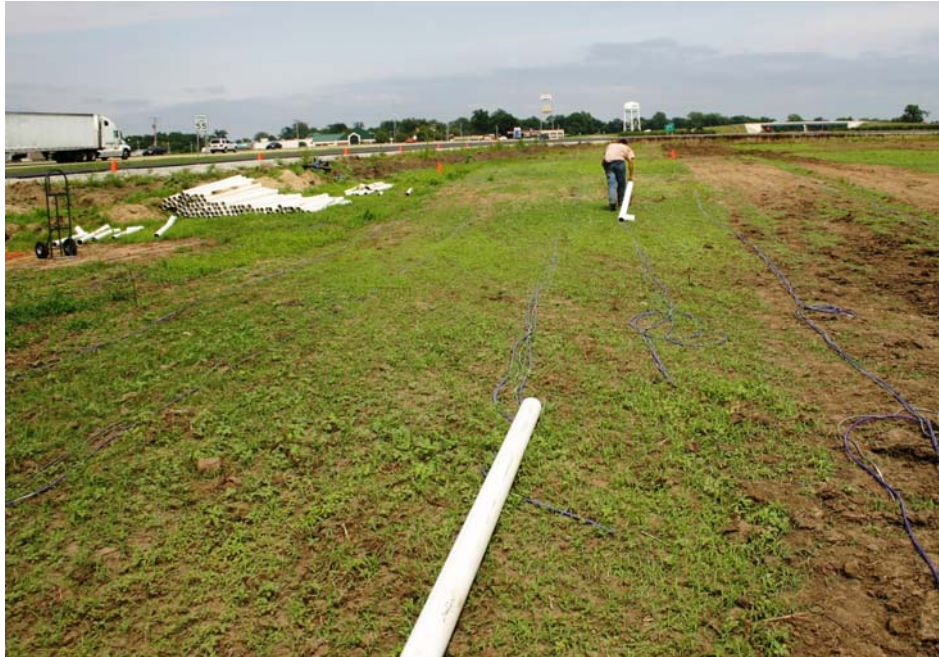
Figure 5.10 – Pipe Feeding Process
