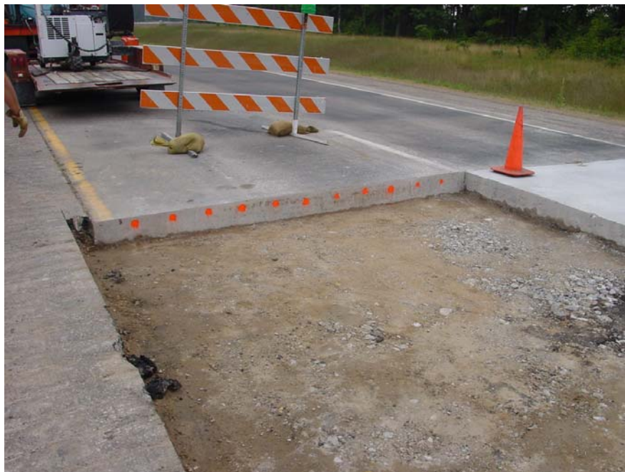
Figure 18. Layout of locations marked for drilling in the existing PCC.
