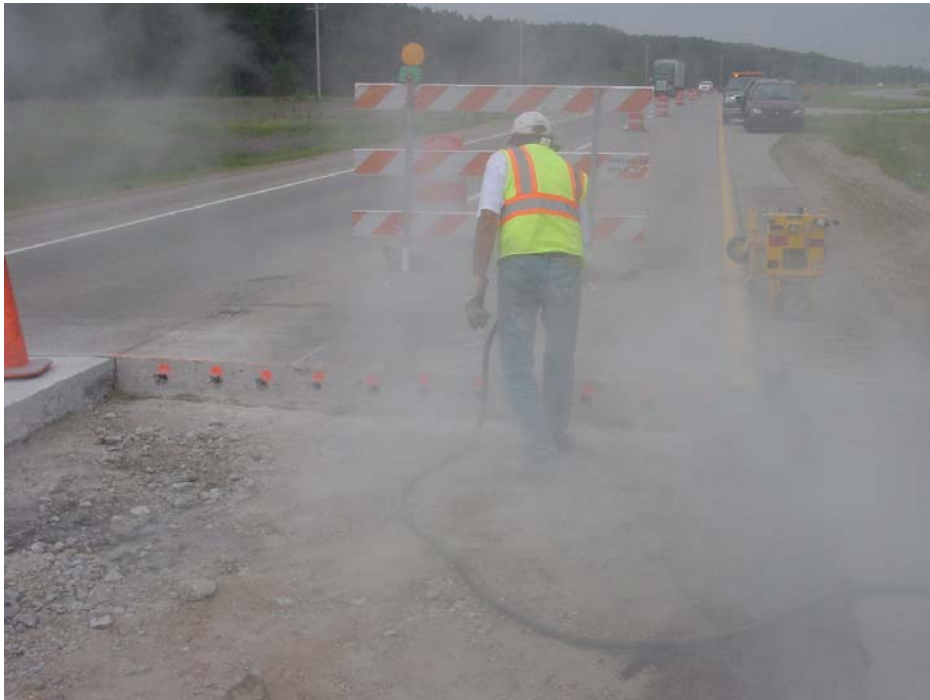
Figure 20. Cleaning drilling dust.
