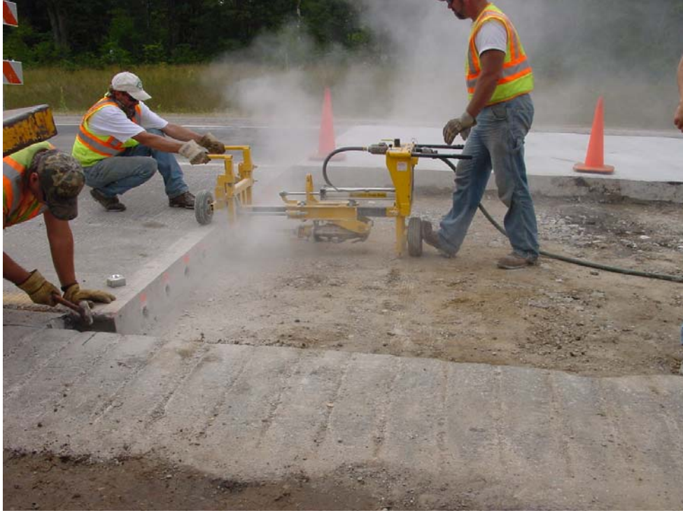
Figure 19. Drilling the existing PCC.
