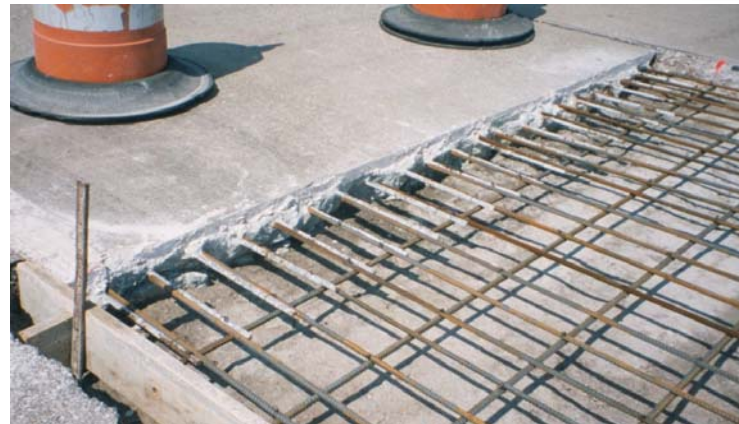
Figure 10. CRCP full-depth repair tied splice details.
