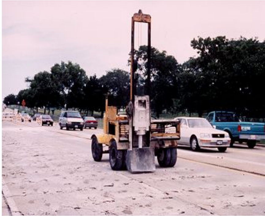
Figure 15. "Light" drop hammer breaks the deteriorated PCC.
