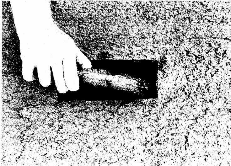
Figure 6—Top view of lifting lug in the timber block insert
