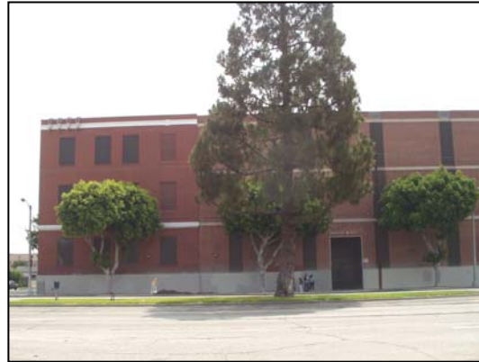
Figure 22. Pacific Bell new building at the east side of Vermont Ave
