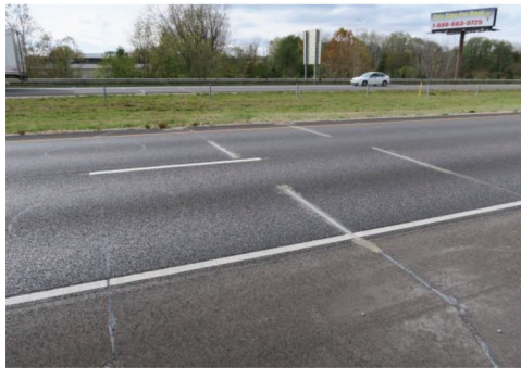
(b) WIM #3700 Physical Components and Condition
