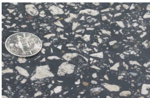
Figure 2.2 Close-up of chip seal with fog seal.
