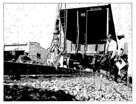
Prototype Rail Uplift Tests for Rail Longitudinal Force Measurement
