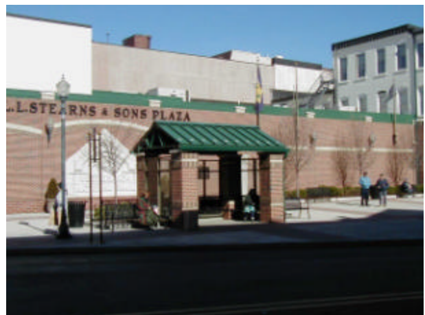
The L.L. Stearns & Sons Plaza, which is part of the Trade & Transit Centre Project, has covered shelters for bus riders.
